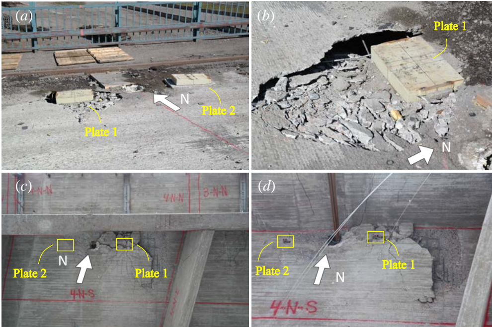
Figure 13. Photos of the failed bridge deck slab after shear failure: (a) & (b) are photos at top of the slab and (c) & (d) are photos at bottom of the slab (Bagge, 2014).
