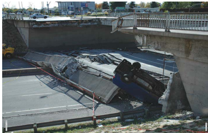
Figure 1. The western part of the collapsed overpass in Quebec, from the eastern abutment, Johnson (2007).
