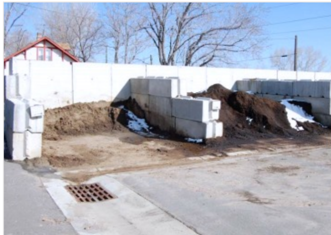
Figure 3.6: Unprotected storage area where the material can pollute stormwater and directly reach the sewers. (Urban Drainage and Flood Control District, 2010)
