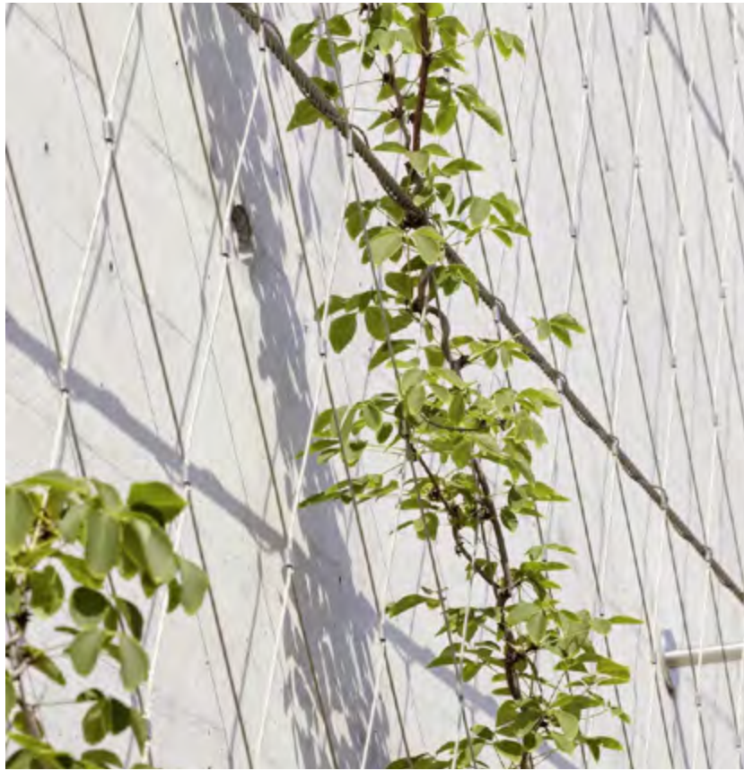
“Webnet” stainless steelwire from Jakob rope systems.
