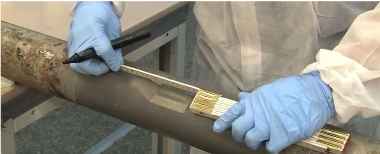
Figure 18 A distance on each side of the damage is marked out to show where the FRP should be applied. The pipe has been prepared with a primer to prevent further oxidation of the pipe(Youtube Woronko premium partner Loctite partner channel, 2014).
