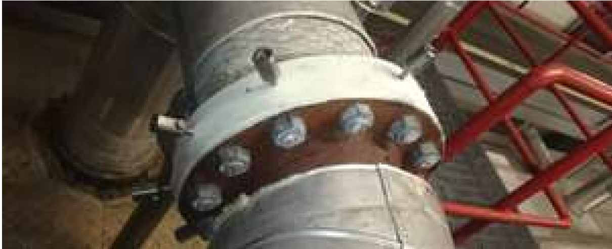
Figure 10 Shows a repair for a flange joining two pipe sections. The valves on the box let the injected compound to cure (SMC Swede, 2016)
