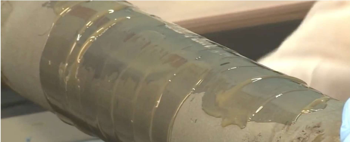
Figure 21 After the epoxy has hardened an adhesive is added (Youtube Woronko premium partner Loctite partner channel, 2014).
