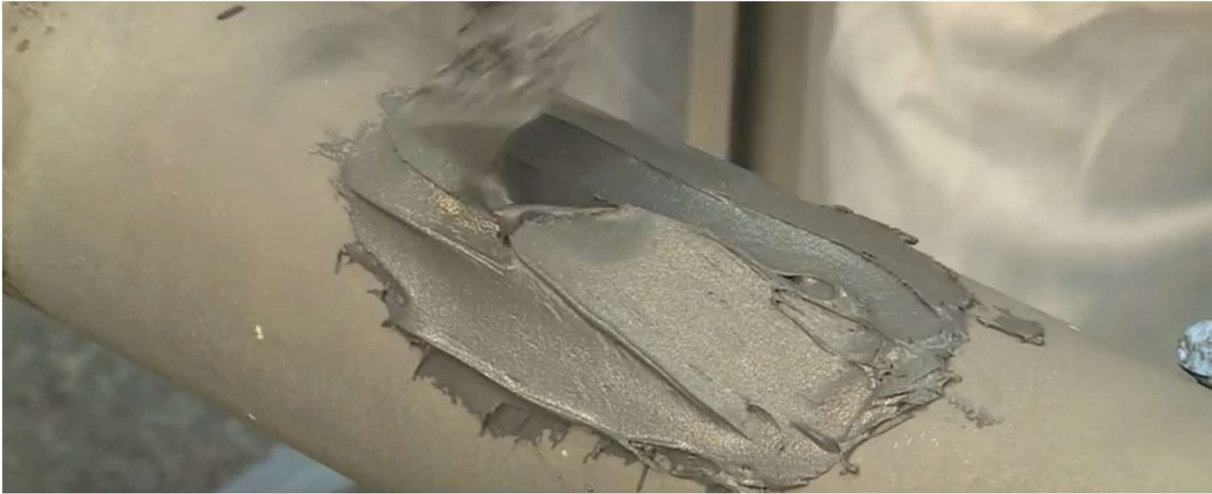
Figure 19 An epoxy is applied to build up the pipes original geometry (Youtube Woronko premium partner Loctite partner channel, 2014)
