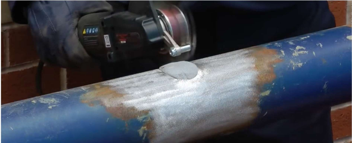
Figure 17 The pipe surface is prepared for wrapping by grinding the pipe material until white metal occur (Belzona Channel, 2011)
