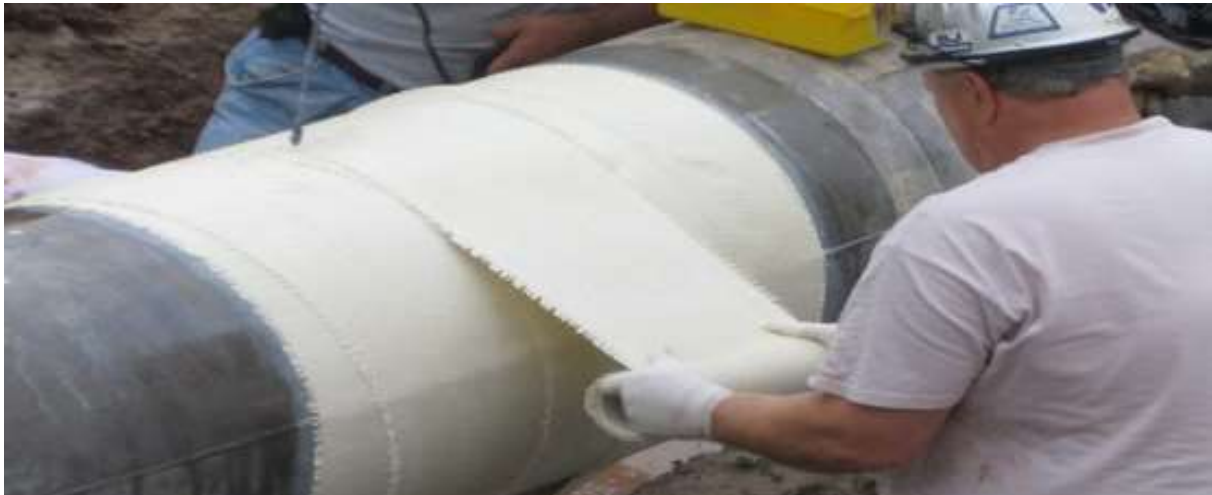
Figure 14 Example of repair with FRP wrapping (Power wrap, 2013)
