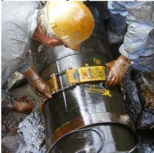
Figure 11 Shows a clamp made of fabric. The method is used for temporary repairs and can be combined with a compound box to increase lifetime (3XEngineering, 2016).
