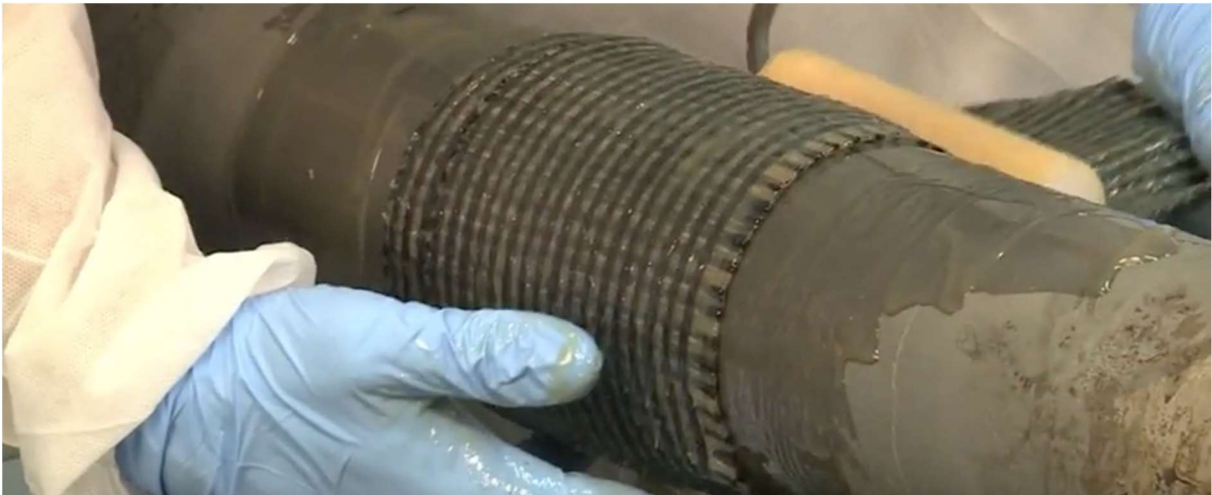
Figure 23 The adhesive attaches the FRP-wrap to the pipe (Youtube Woronko premium partner Loctite partner channel, 2014).
