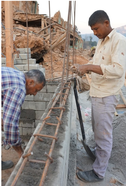
Figure 18. The construction of a tie beam at sill level in Majhi Gaun.
