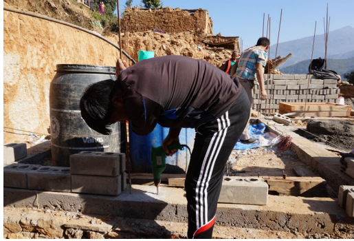
Figure 6. Drilling holes for anchorage of rebars.
