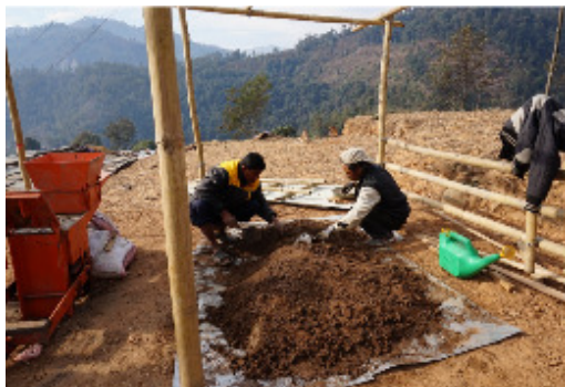
Figure 3. Mixing cement and soil in Majhi Gaun
