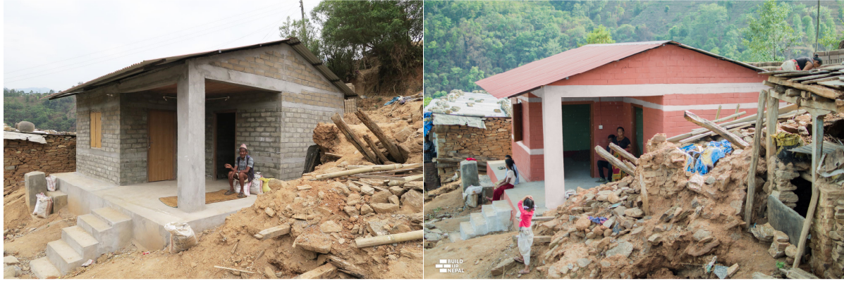
Figure 22. CSEB building in Majhi Gaun before and after painting.
