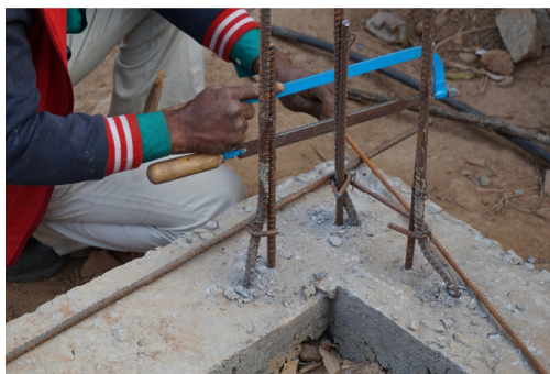
Figure 5. Bent rebars in Majhi Gaun
