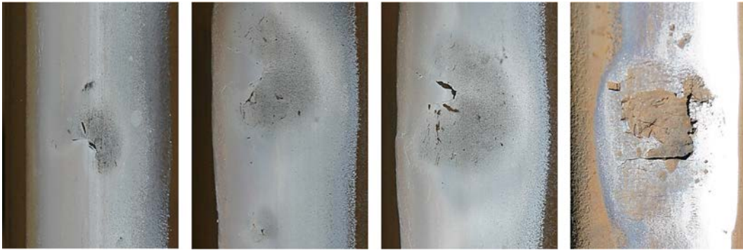
Figure 2. Examples of squats of different severity in field, as well as an example of spalling (far right).
