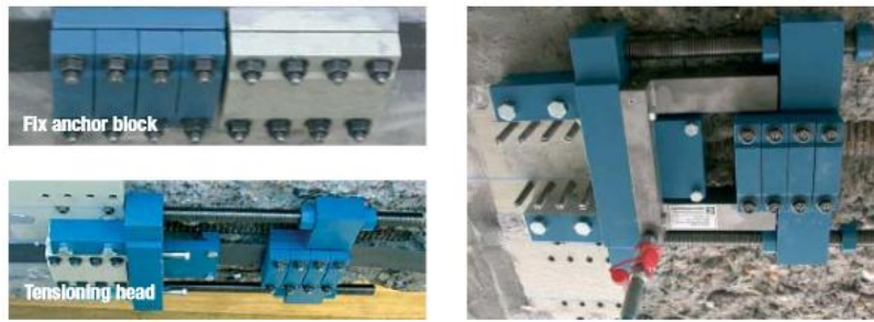
Figure 4.8 Tension head with temporary anchors and permanent anchor block from the Sika LEOBA system [36].
