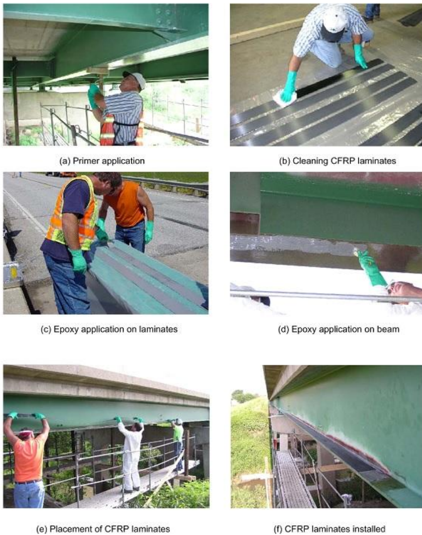
Figure 3.8 Preparation and installation of CFRP laminates on a steel beam [9].
