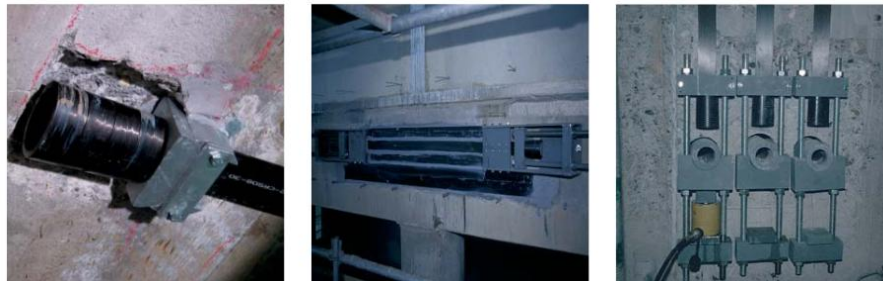
Figure 4.9 To the left is a picture of the Sika StressHead system installed with the permanent mechanical anchor locking the StressHead in place, and to the right is two pictures of the steel framework [36].
