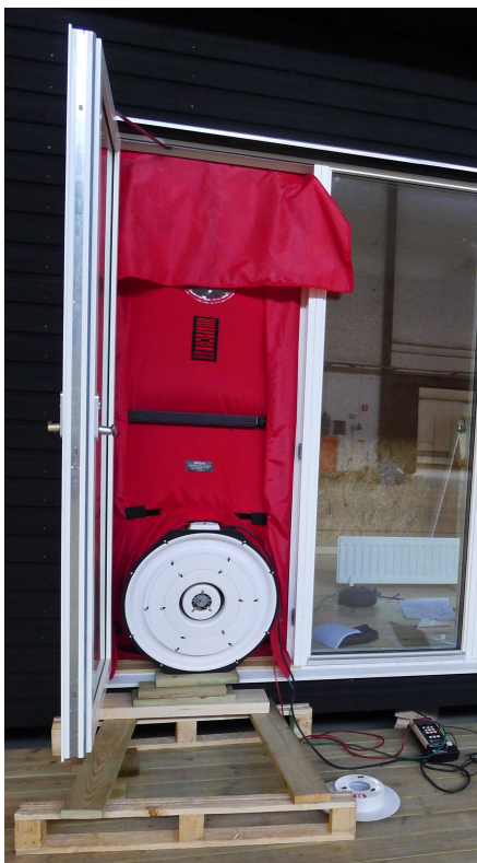
Figure 15: Blower door equipment mounted in the guesthouse.
