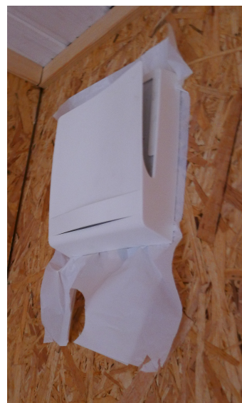
Figure 16: Ventilation duct sealed by squeezing a plastic sheet behind the ventilation cover.
