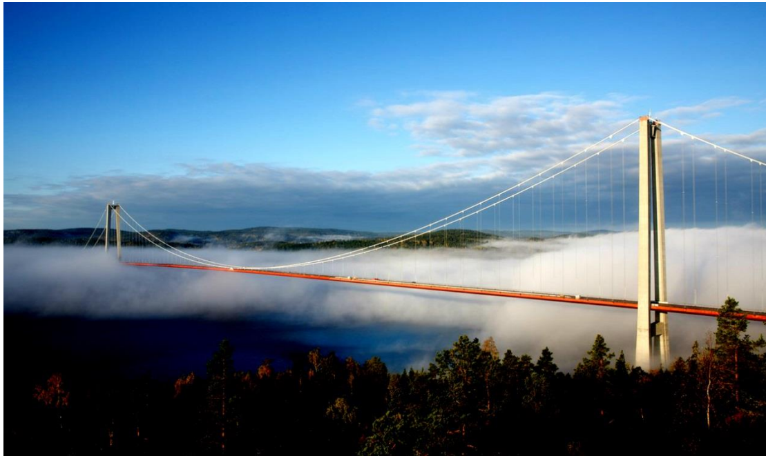
Figure 3.1 Höga Kusten bridge ( http://www.bridge-info.org ).
