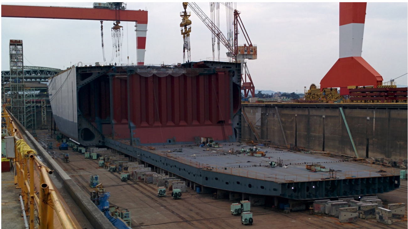
Figure 14. A 500 meter long bulk ship is being assembled in Hiroshima, Japan.
