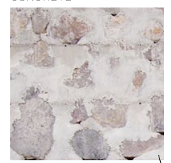
WHITE CONCRETE WITH CAST IN NATURAL ROCKS
