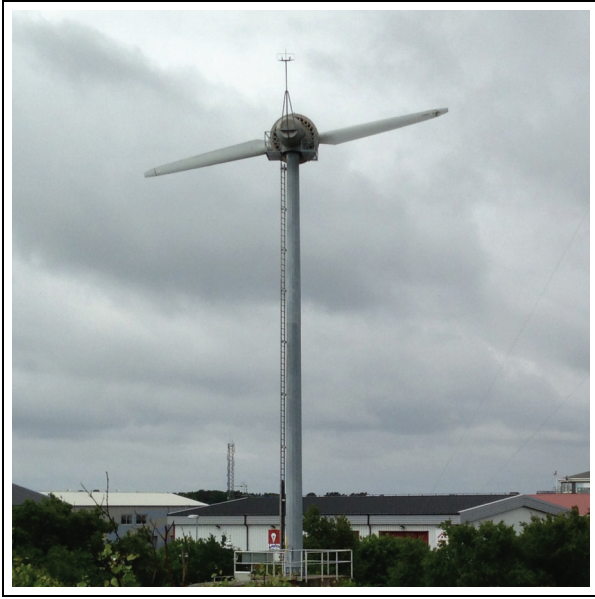
Figure 1. The Höno turbine located outside Gothenburg, Sweden. The turbine has two blades with rotor diameter 13.5 m and power rating 35 kW. The turbine parameters are summarized in Table 1.
