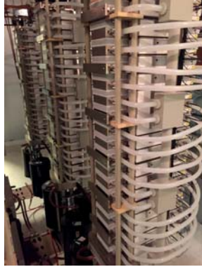
Figure 7.3: Voltage source converter. IGBT stacks for the 10kV converter.
