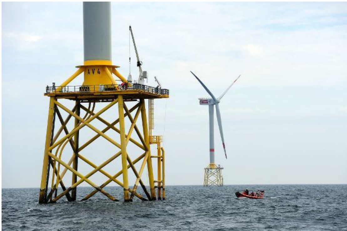
Figure 3.2 Jacket structure (Crampsie 2014)
