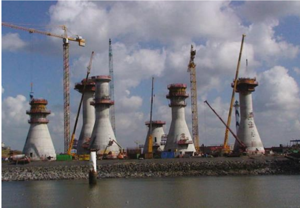
Figure 3.3 Gravity base foundations (Kaiser and Snyder 2012)
