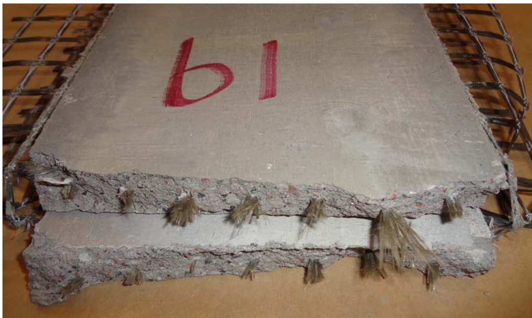
Figur 5-2 The condition of a plate with basalt textile and concrete mixture 1 after failure.
