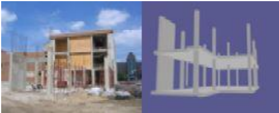
Figure 2.10 Comparison of 3D model with actual image using Augmented Reality (Fard & Mora, 2007:4)
