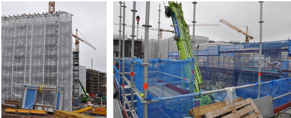
Figure 4.4 Construction site 3,4 and 5
