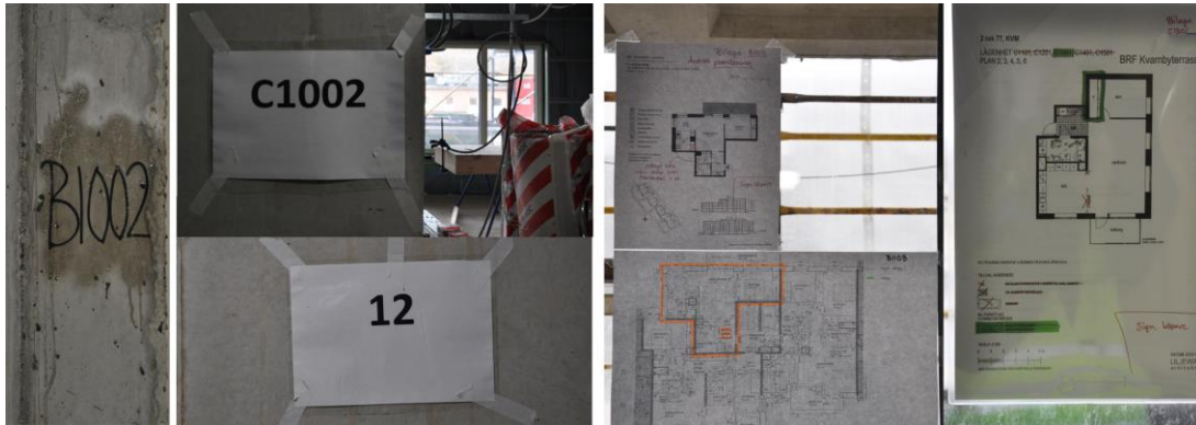
Figure 6.6 Markings on wall (on left) and 2D drawings with specification (on right)
