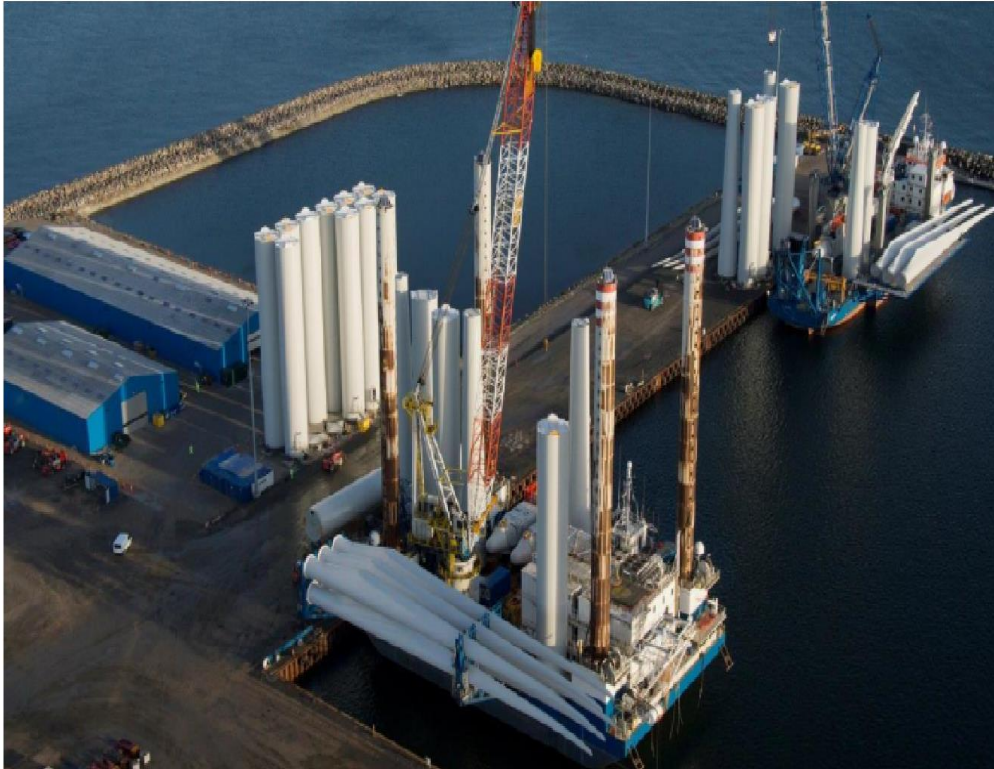
Figure 15: Loading turbine components (Source: DONG Energy 2016)
