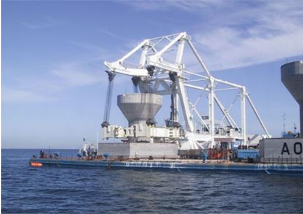
Figure 8: Installation of foundation (Source: http://www.tech-marine.dk )
