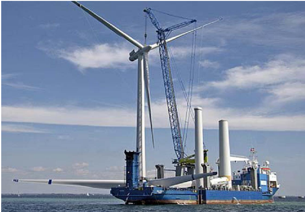
Figure 10: Turbine Installation (Source: Vattenfall, 2008)
