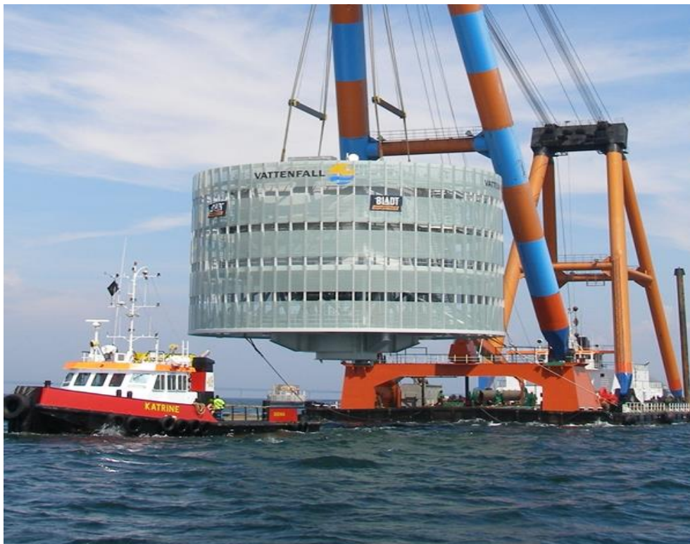
Figure 11: Substation installation (Source: http://www.bladt.dk )
