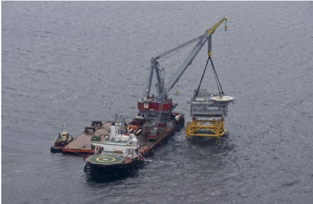
Figure 17: Lifting and installation of Anholt substation (Source: Energinet.dk)
