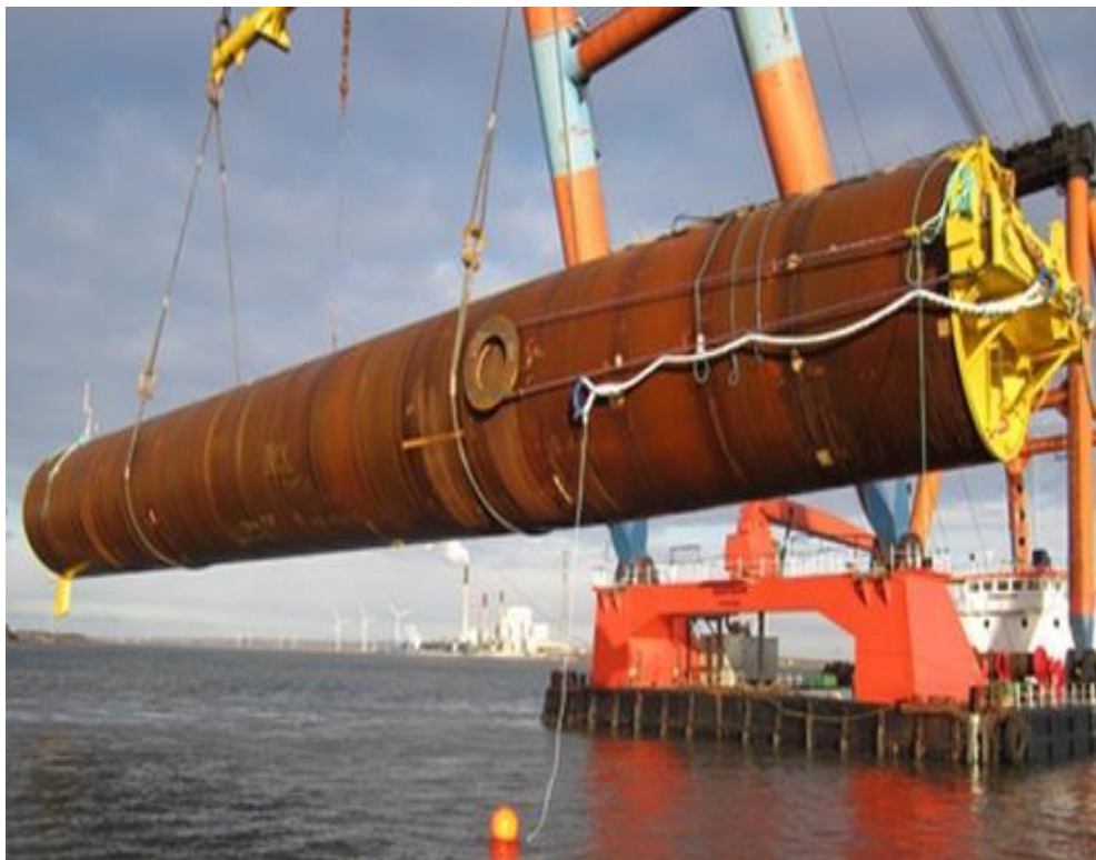
Figure 13: Lifting monopile at Grenaa (Source: DONG Energy 2016)
