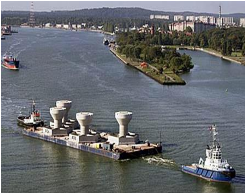
Figure 7: Transportation of foundations (Source: Vattenfall, 2008)
