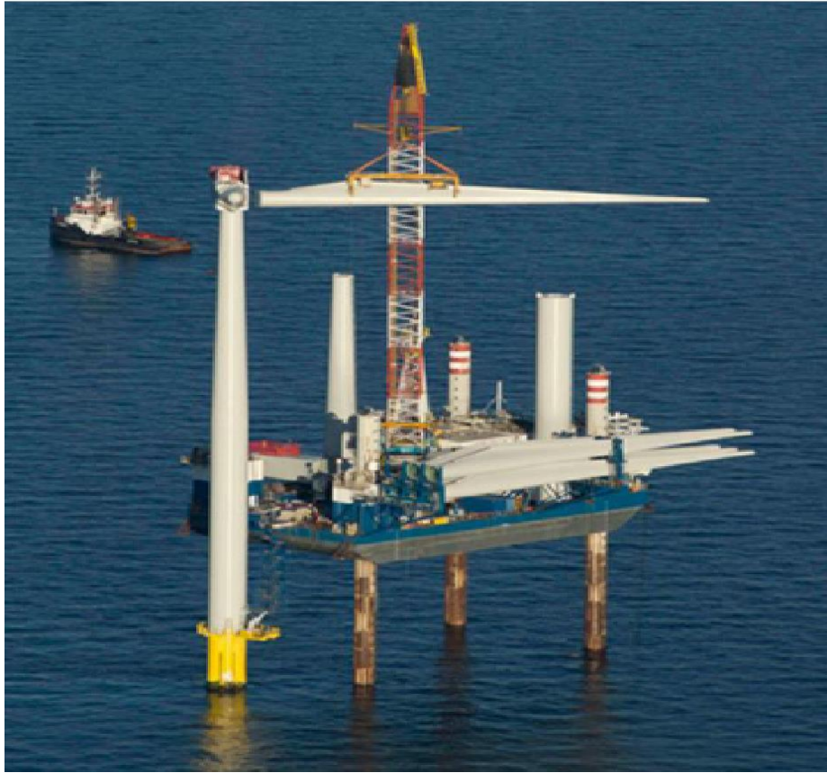
Figure 16: Installation of turbine components (Source: DONG Energy 2016)
