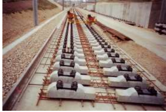
Figure 5 Ballast-free tracks/Slab tracks (Terfloth, 2004).
