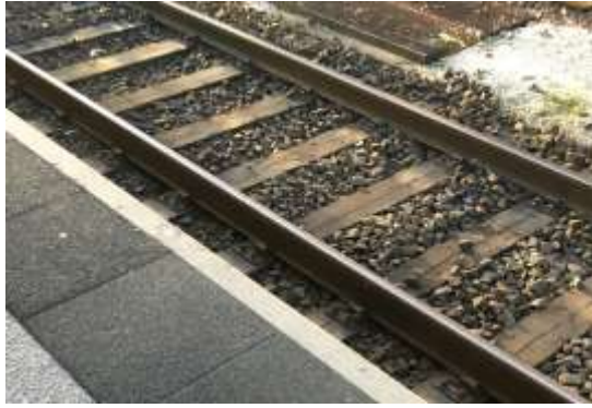
Figure 4 Conventional railway with ballast tracks.
