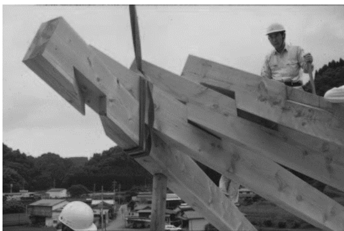
Figure 4.15 Notched Vatariago connections for Seiwa Exhibition hall. [14]
