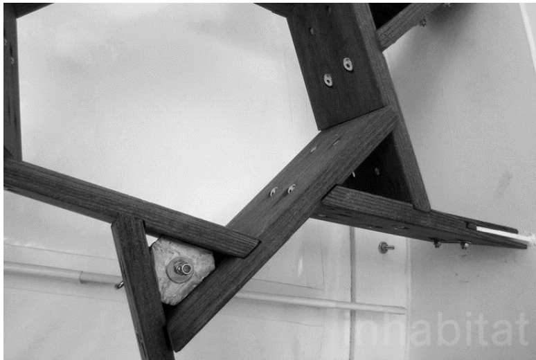
Figure 4.11 Bolted connection in Kreod Pavilion. [12]
