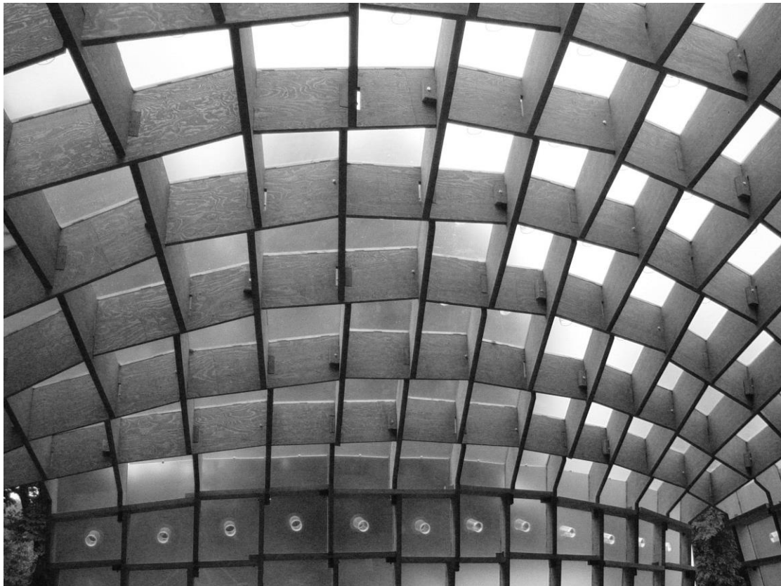
Figure 2.6 Zollinger-like connections in Alvaro Siza's Serpentine Gallery [5] Pavilion.
