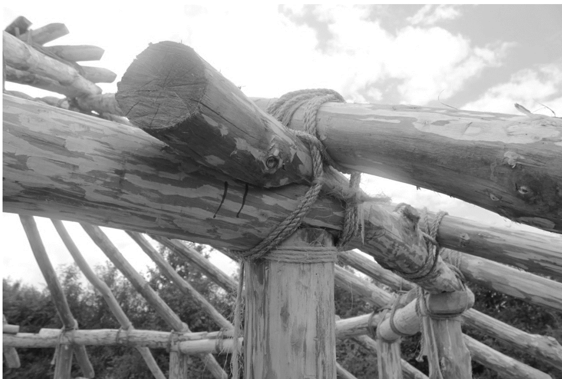
Figure 4.7 Lashed joint of a Roundhouse in France, using jute rope. [10]
