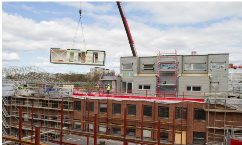
Figure 2 - The production of the new added floors in Tegeludden (Moelven, 2016)
