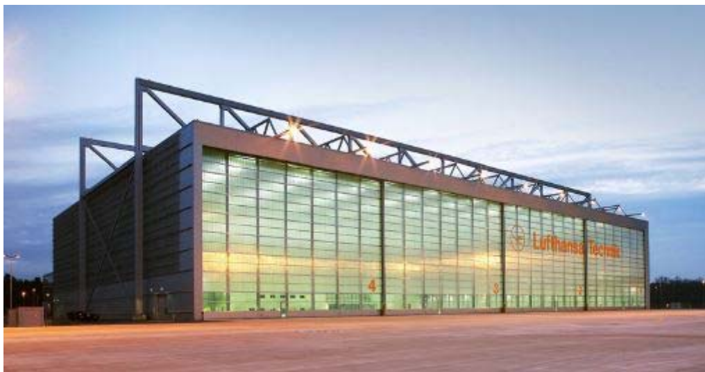
Figure 2.11 Airbus hangar at Frankfurt Airport (Willms, 2009).
