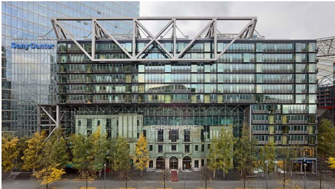
Figure 2.12 HSS truss girders in Sony Center building F, Berlin (Anon., 2016).
