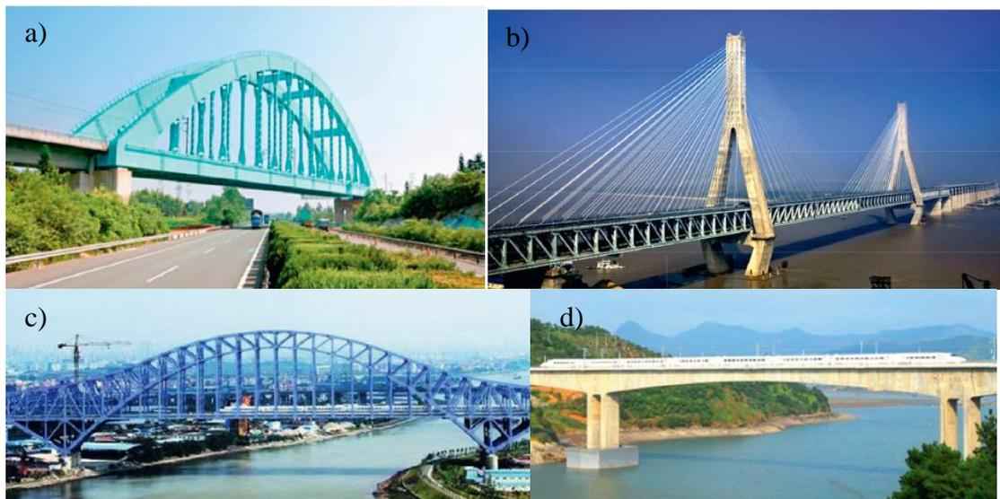
Figure 3.12 Railway bridges in the Chinese high-speed network for medium and long spans. a) Tied steel arch bridge (Tingsihe Bridge, main span 140 m), b) Cable-stayed bridge with truss girder (Tianxingzhou Bridge, main span 504 m), c) Steel truss arch bridge (Dongping Bridge, main span 242 m), d) Rigid frame bridge (Tianluo Bridge, main span 160 m) (Dai, et al., 2014).
