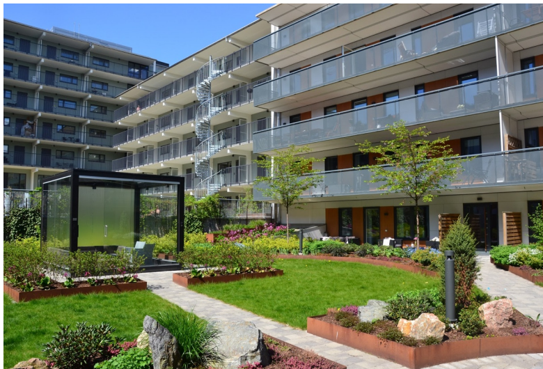
Figure 5 - View over the garden house and the balconies to the right. (The house behind the garden house is another project).
