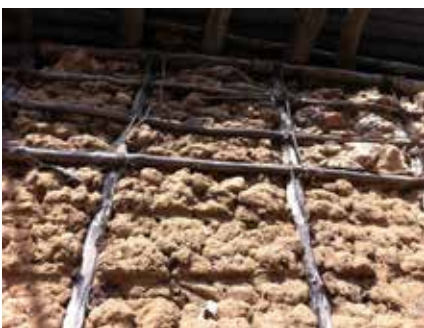
Wall made by wattle and daub
