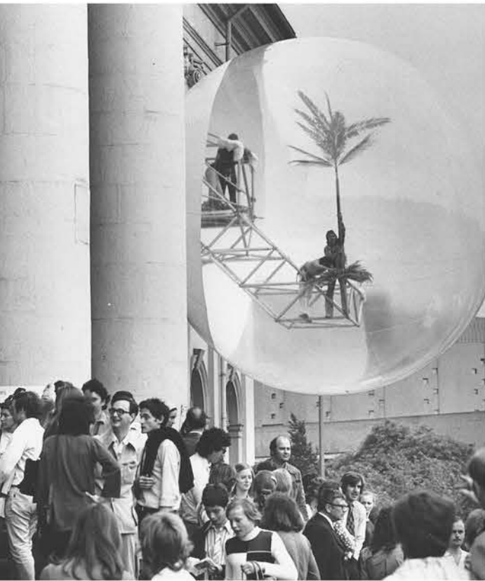
fig.16 Haus Rucker Co created a space for relaxation and play with an inflatable structure on the façade of an existing building. This is also an example of how a space frame at certain points can penetrate the inflated plastic.
