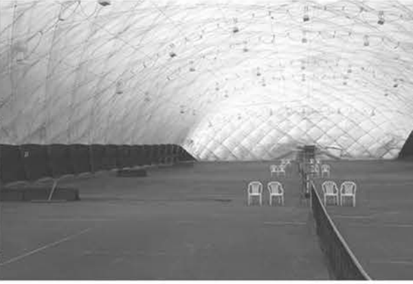
fig.15 Large inflated tent covering a tennis hall. The structure is withstanding the winds of an unprotected field.
