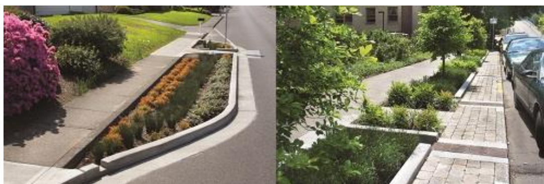
Figure 2.3 Two types of rain gardens in Portland: curb extension (left) and a so called green street (right) with small rain gardens in the pavement (Source: City of Portland, 2016).
