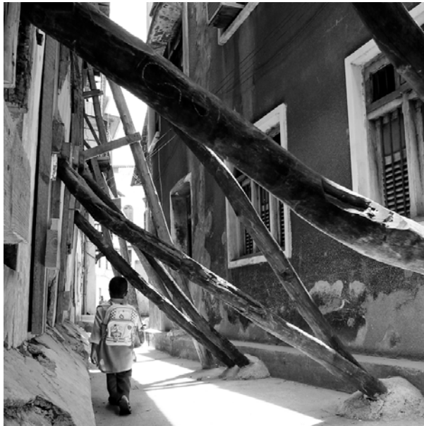
Braced walls of collapsing house.
