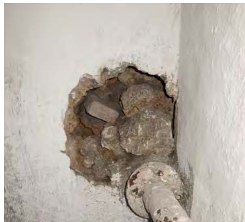
11 a. Pipe from cold pool to runnel (seen from urinals).
