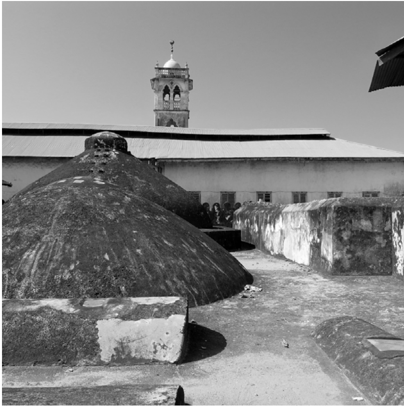
The 400 sqm roof, looking towards Hamamni Street, with the dome over the warm room closest by.
