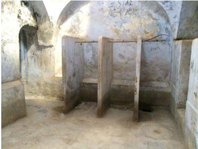
The retrofitted showers with concrete partitions.
