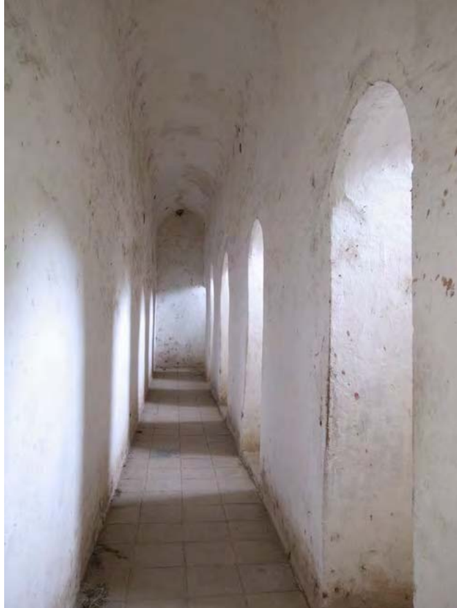
All but the public hammam in Stone Town feature a row of five pit latrines. These are the ones in the baths at Maruhubi where there is also a row of five separate baths in combination with the Persian style hammam.
