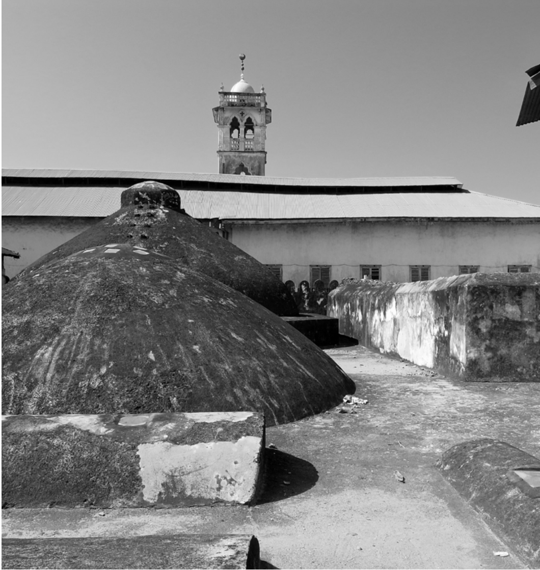
Rain water collecting roof with the the large cool room dome seen furthest away.
