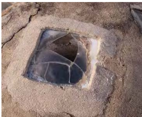
Many of the existing panes are broken.
