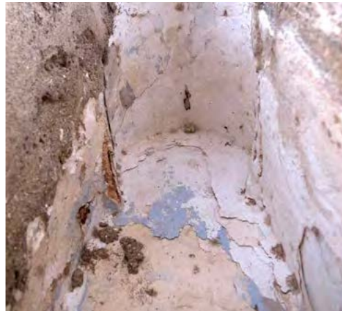
Decorative exterior niche by entrance. Note the blue layer.
