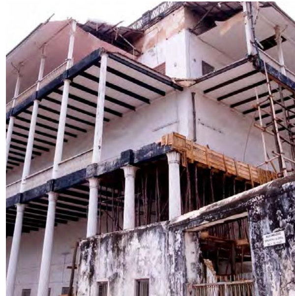
The House of Wonders under restoration since long.
