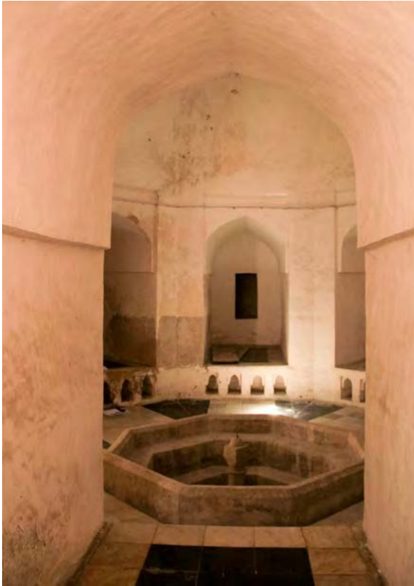
Above: The first room of the hammam, the cool resting place to return to after exhausting the body in hot rooms. Note the two original colours of plaster visible where paint has fallen of in the middle of the picture.
