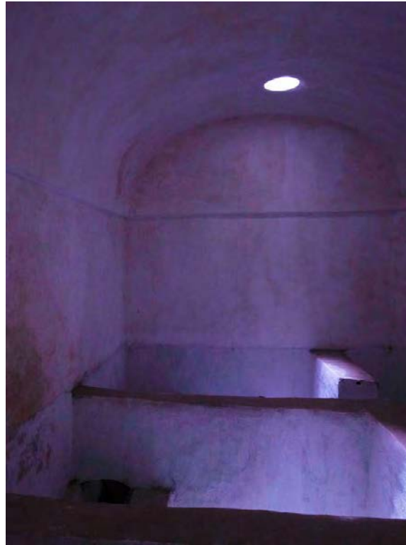
Lighting using the same light shafts as for daylight, only now with spotlights mounted on top of the shafts.
