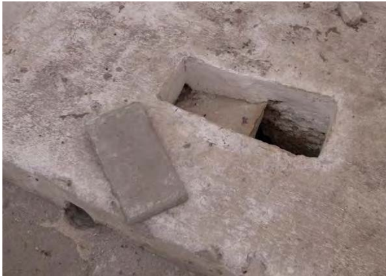
Pit latrine with slanted tile and drain connected to the same outlet. Reminiscent of modern urine separating toilets.
