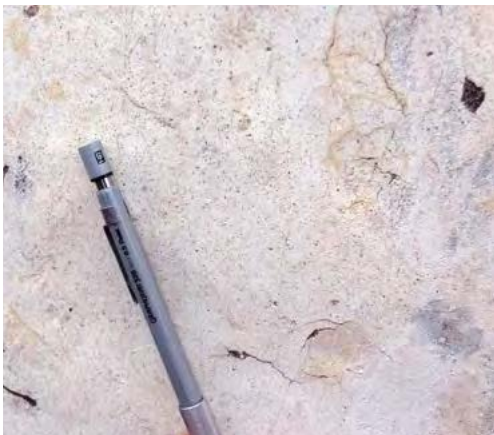
Close up of original exterior plaster
