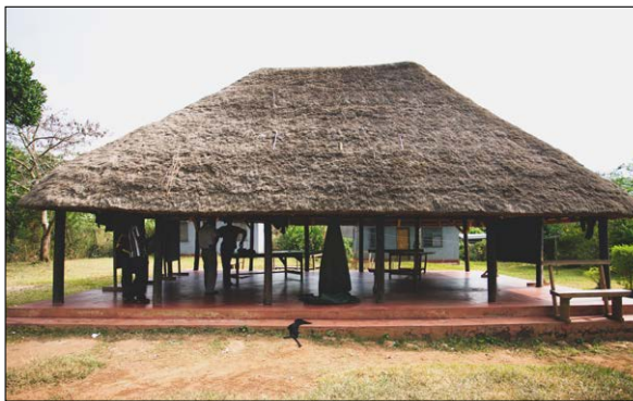
A construction made of poles and banana leaves. The space is used for studies and other activities.
