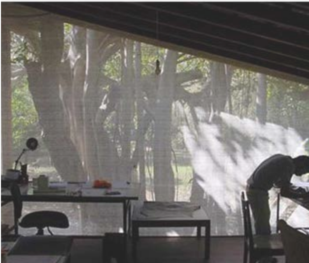
Figure 20: Mumbai Studio uses a thin metal net to keep indoor protected against mosquitos while letting airflow and light enter the building.
