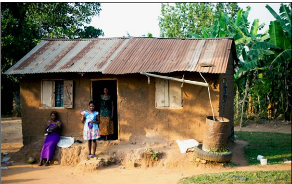
Modern rural structure The houses are rectangular and usually made of bricks and mud, covered with an iron sheeting as a roof.
