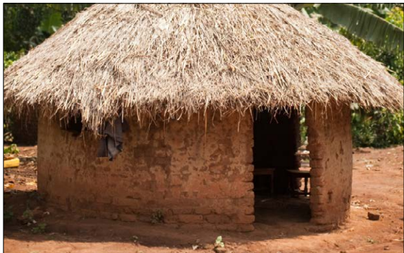
Figure 29: Traditional hut. Traditionally the village structures are round and made of clay or bricks with a straw roof.
