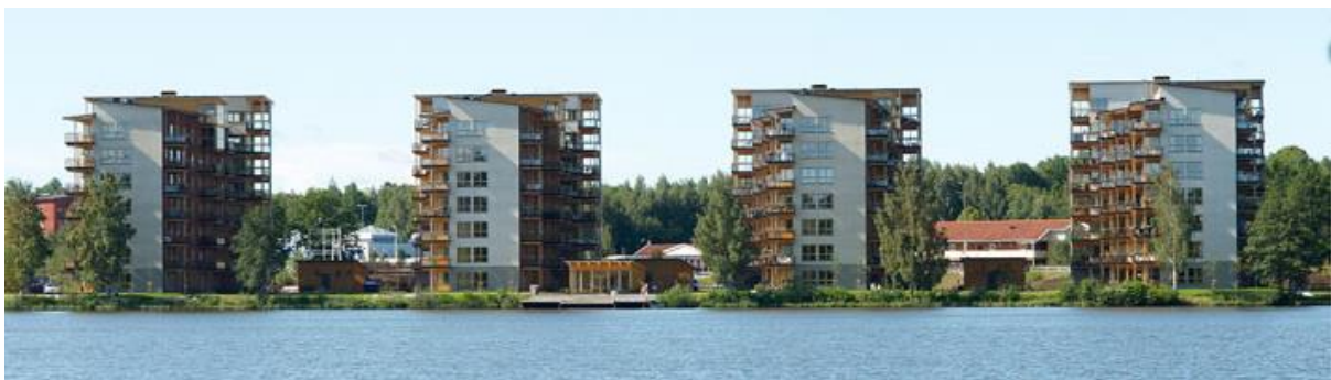
Figure 24: Project Limnologen in Växjö (Midroc Property Development AB, 2016)
