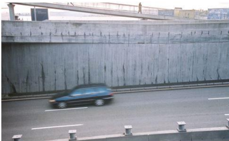
Figure 2.8 Through cracking as an effect of external restraint (Bjøntegaard 2011).
