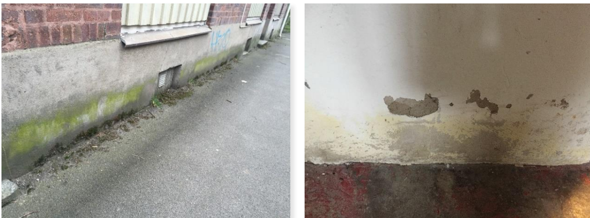
Figure 20 Biological growth in external and internal walls (Source: personal archive)
