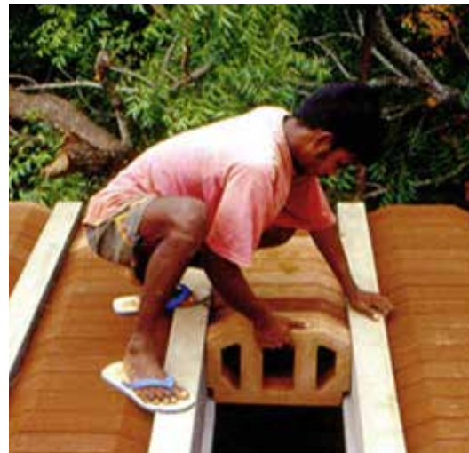
Construction of hollow roof with hourdi blocks Source: Auroville Earth Institute 2016
