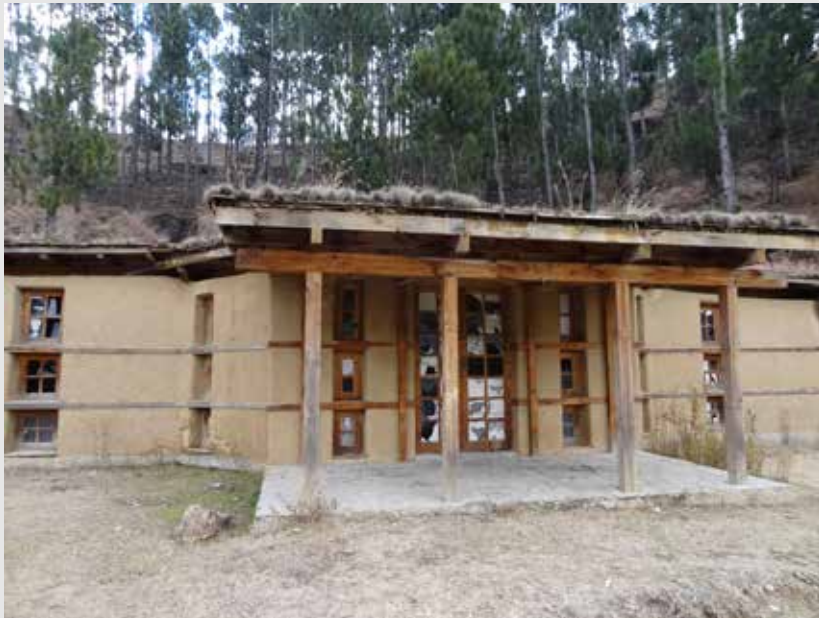
This heritage house was designed by Yasmeen Lari and built to demonstrate to the locals how they could use traditional materials and techniques today.
