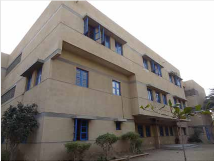
Schools in Karachi are built with plastered concrete blocks. Pigment is mixed in with the plaster to eliminate future need for repainting.
