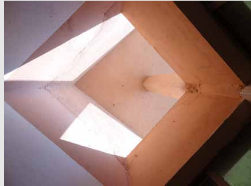
This decorative modern windcatcher shows that windcatchers can also let in diffuse daylight.
