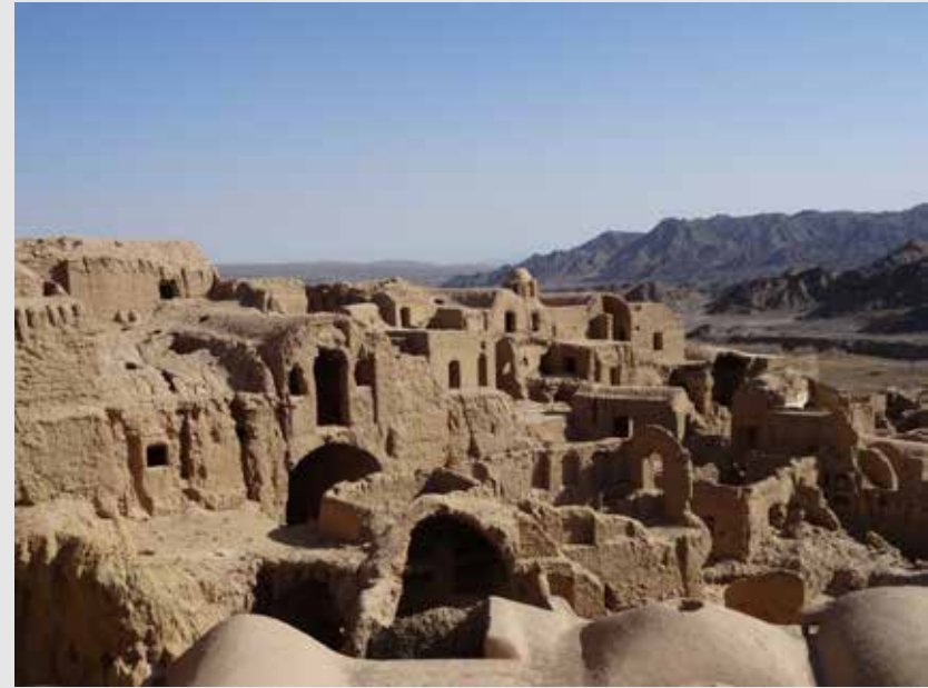
The houses in Kharanaq, Iran are clustered together to provide protection from dusty winds and to minimize the area exposed to solar radiation.
