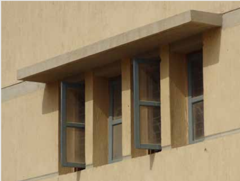
Schools in Karachi and Lahore have shading devices that are designed to block the sun during the summer and let it in during the winter.
