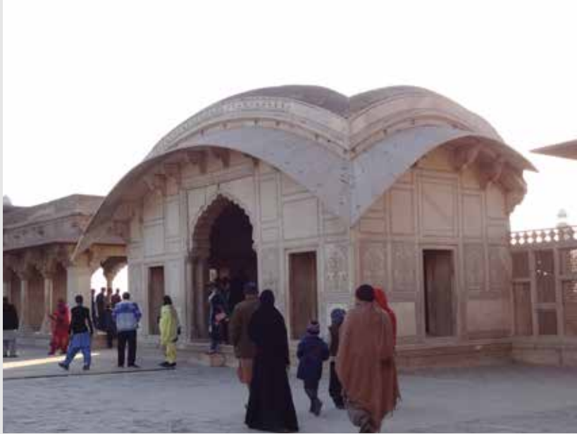
Mughal architecture often includes roof overhangs, which protects the walls from rain and also shades the walls.
