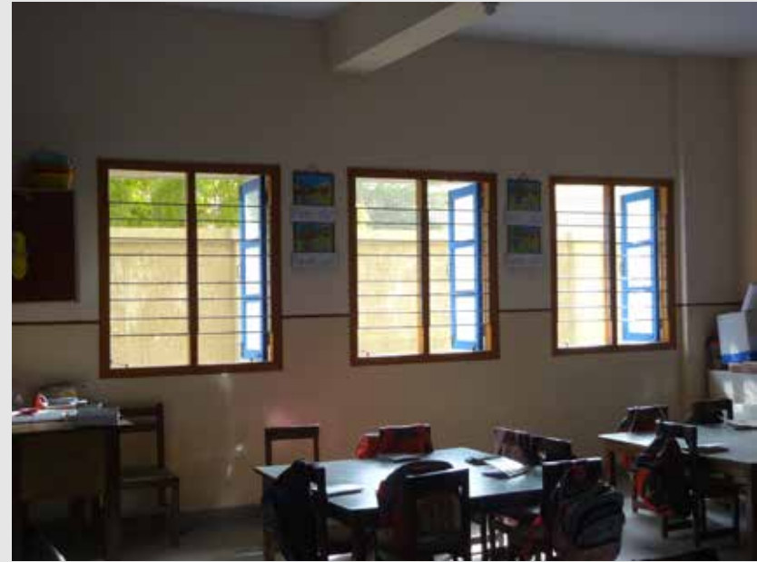
TCF schools rely on cross ventilation through windows, but this often doesn't work as intended.
