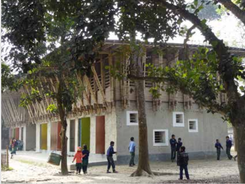
METI Handmade School revived the local villagers' interest in earth buildings by using the traditional material in a new and improved way.
