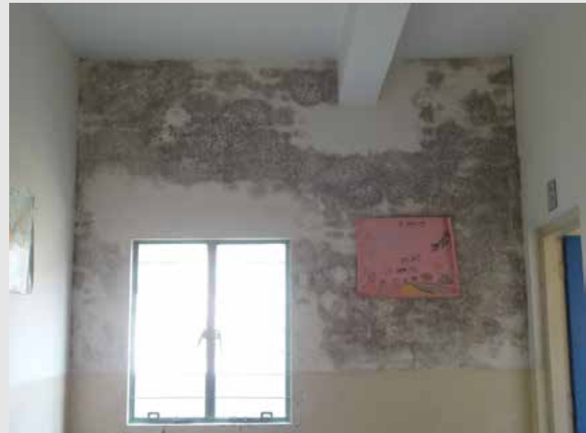
Low-maintenance materials are a high priority for TCF. Some existing schools suffer from severe moisture problems which is a major cost for TCF.
