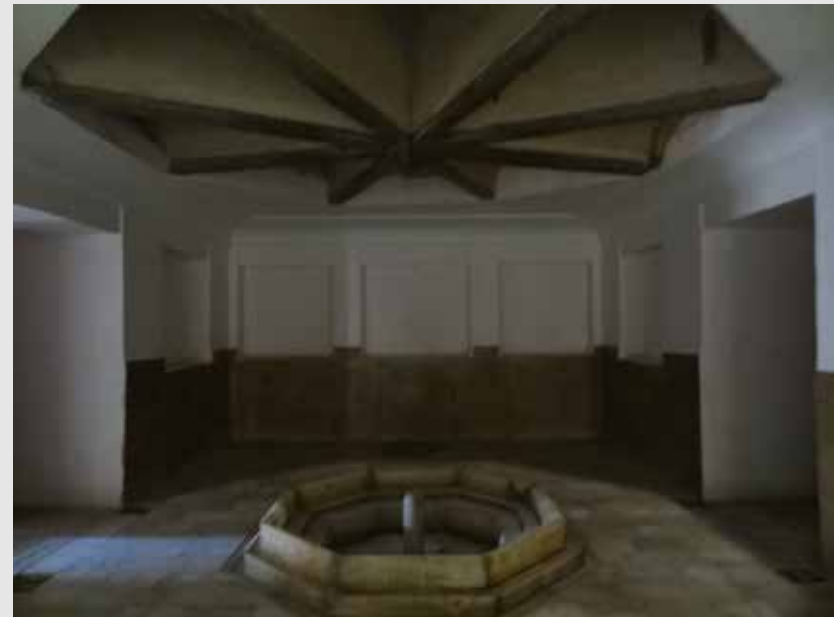
This fountain is located under a windcatcher, and the water cools down the incoming air through evaporative cooling.
