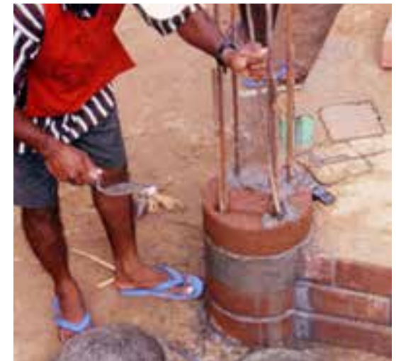
Construction of composite column Source: Auroville Earth Institute 2016
