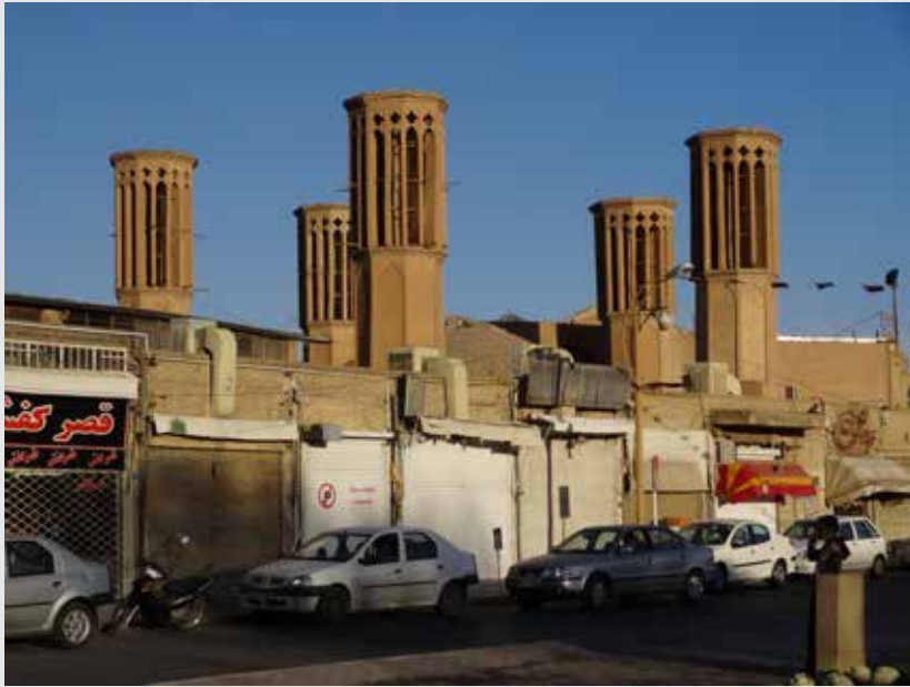
Iranian windcatchers usually have several vertical shafts with openings in different directions.
