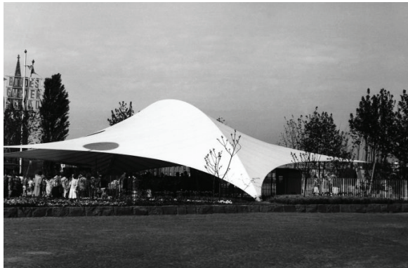
In membrane structures support axes yield strong effects on the aesthetics, this strong relationship between form and function creates a readable design Entrance Federal Garden Exhibition (1957) by Frei Otto
