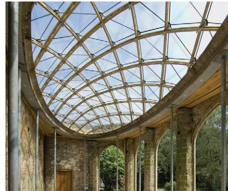
Structural optimization of gridshells can absorb main axes in a shape for efficiency adding aesthetic logic in the process Chiddingstone Gridshell (2007) by Buro Happold
