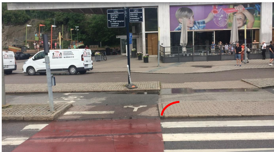
Figure 39 Adjustments of kerbstone to make the turn less sharp.
