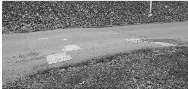
Figure 7.1: A typical round-topped speed bump with a height of 6 cm and a length of 2 m .
