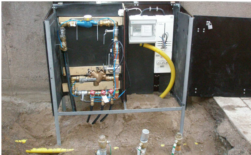
Figure 7 Infiltration utility under construction in central Stockholm. Three infiltration wells (foreground) and cabinet for regulation of infiltration flow. Photo: COWI AB.
