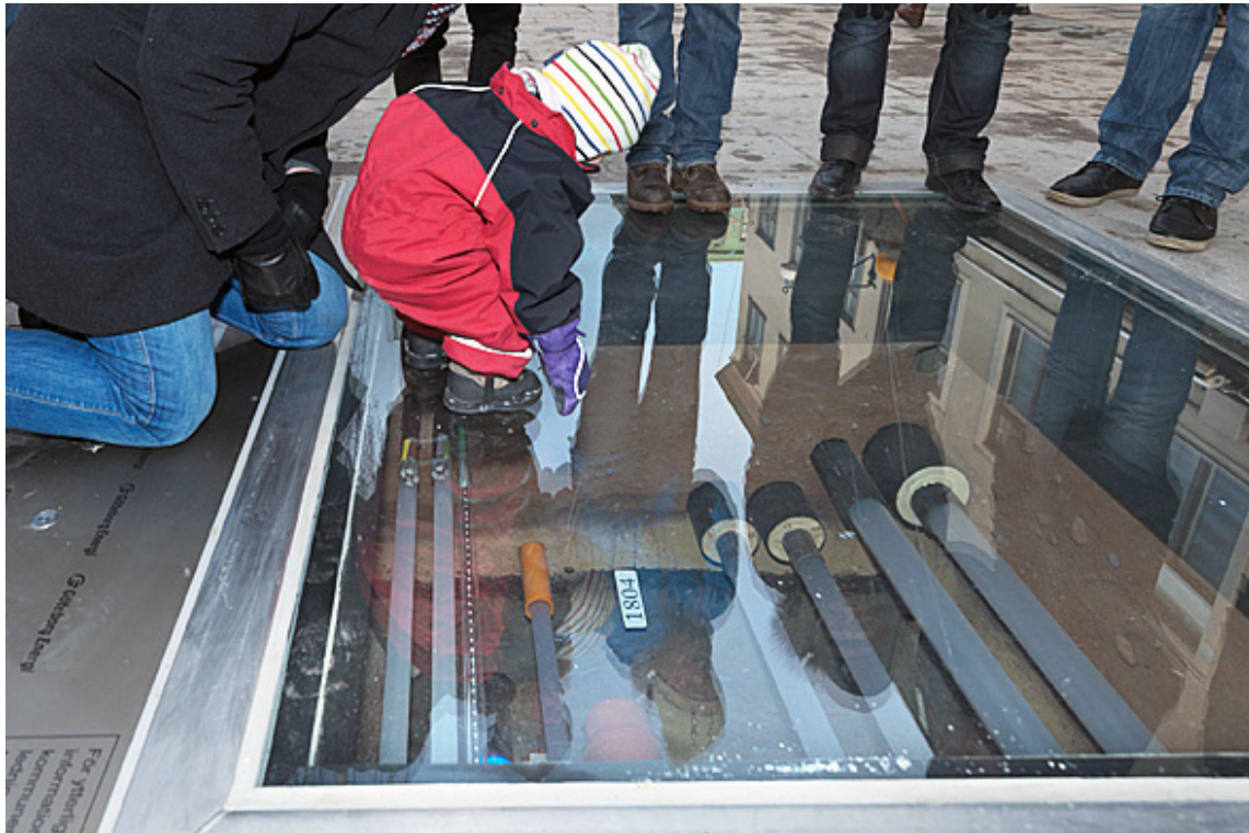
Figure 3. A removed section in the street exposing underground pipes on a street in Gothenburg (photo: Göteborg Energi)
