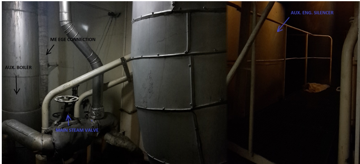
Figure 8: Auxiliary boiler location, Stena Forecaster
