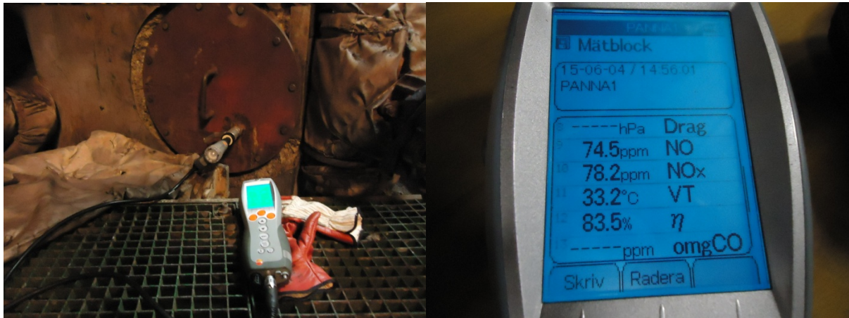
Figure 10: Testo 330-1 auxiliary boiler efficiency result
