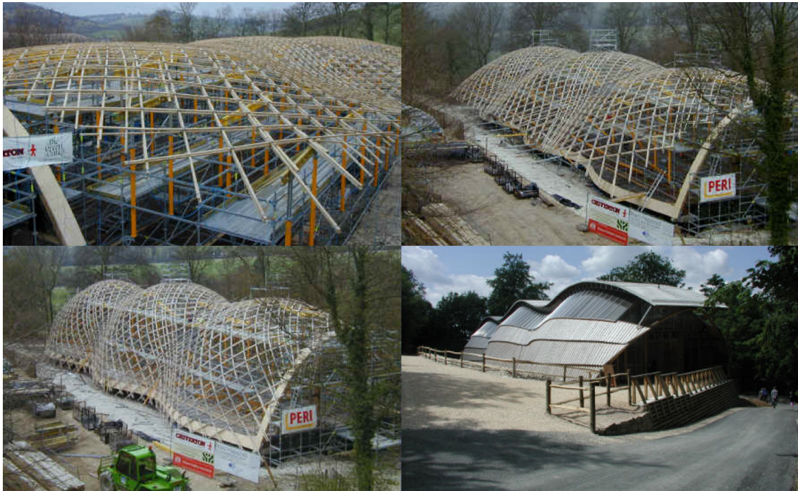
Figure 1.6: The forming process of Weald and Downland gridshell [14]
