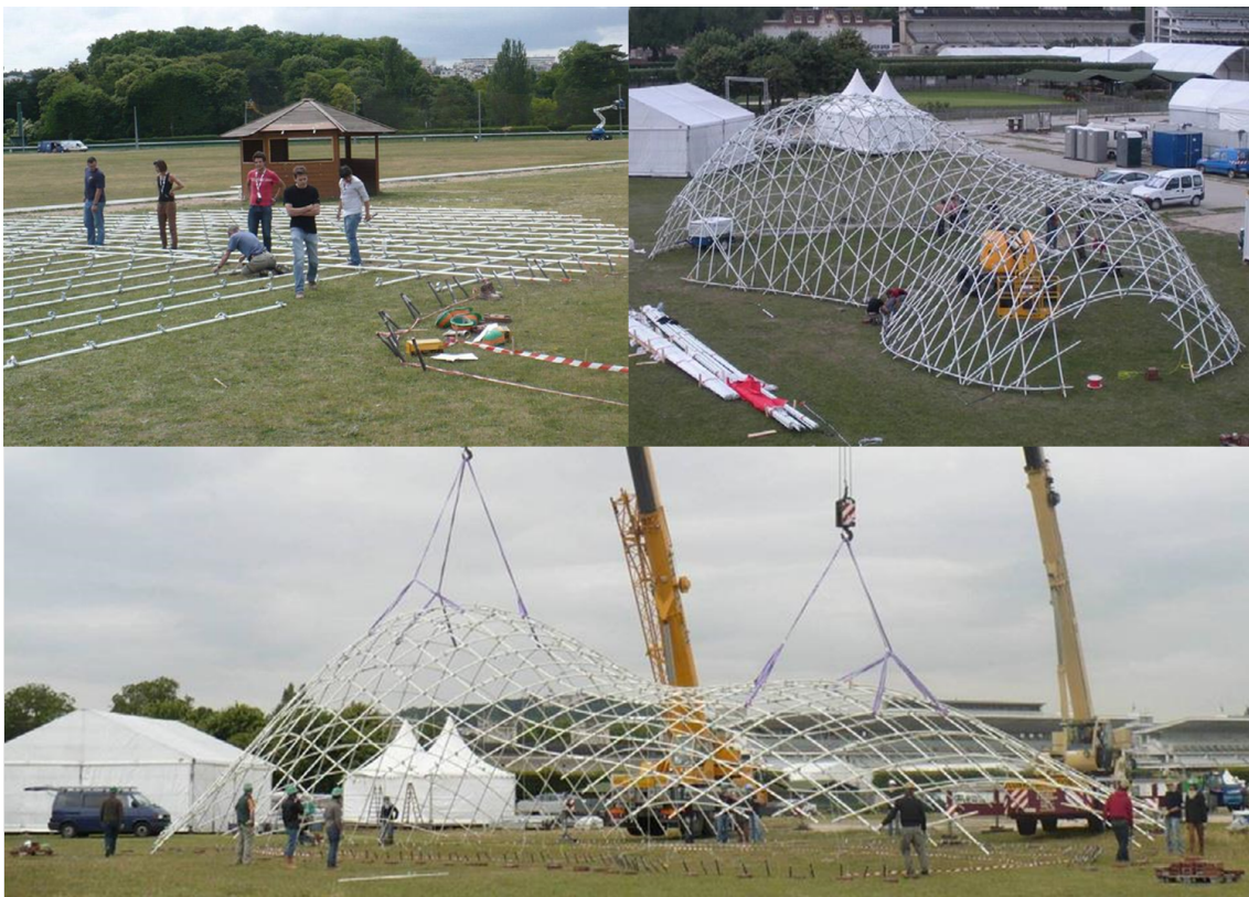
Figure 1.7: Erection process for the Soliday pavilion [13]
