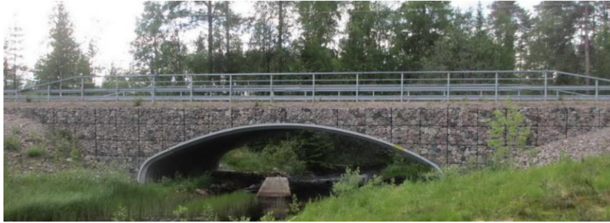
Figure 5.2 Box culvert bridge over Siktån at Rörbäcksnäs (Picture from BaTMan, bridge number 20-1335-1)
