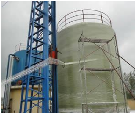
Figure 4.6 On-site filament winding of FRP tube with large diameter [29]
