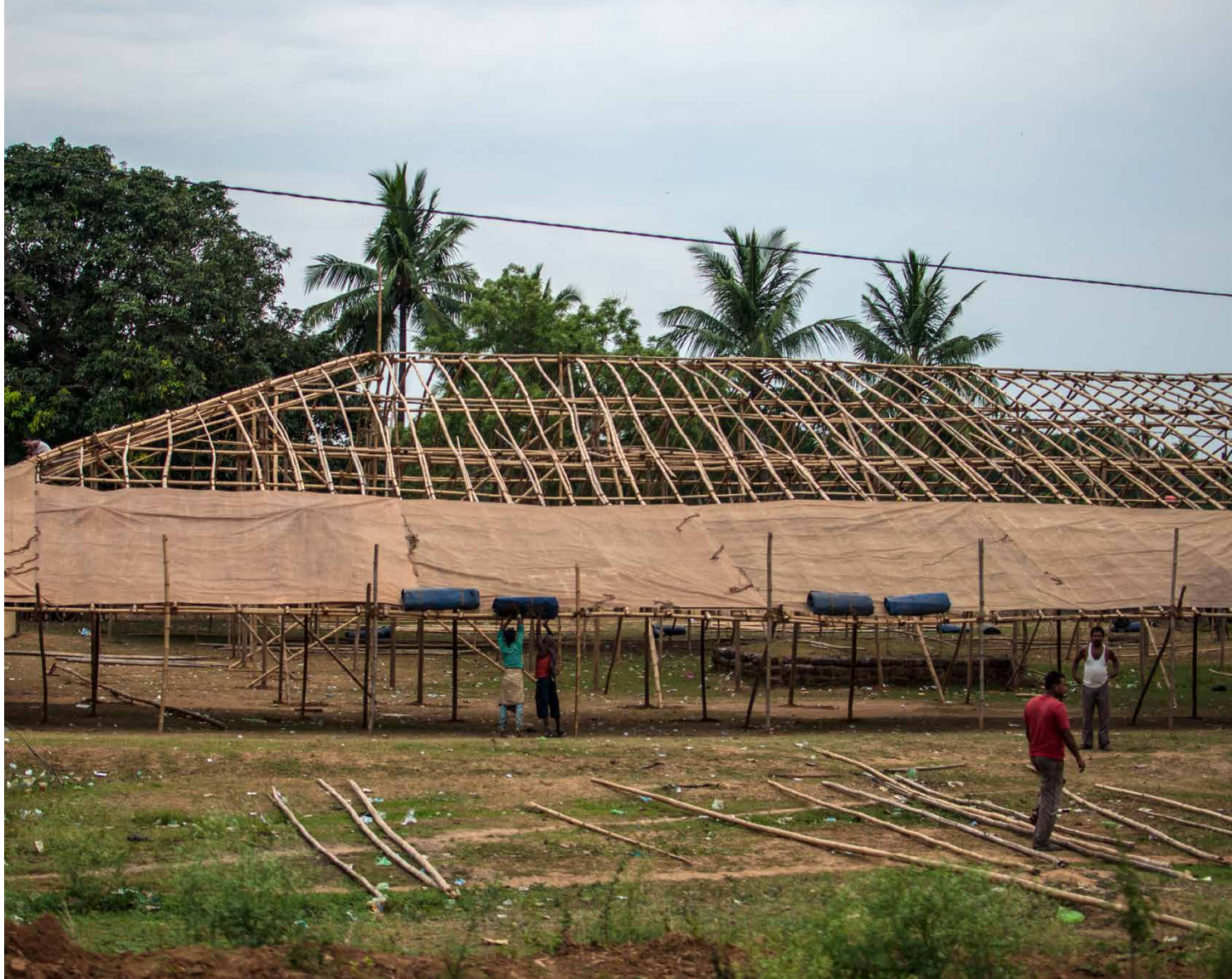
Fig.24 Bamboo is used for the construction of temporary structures, like celebration tents for weddings, Odisha. Photo: AK
