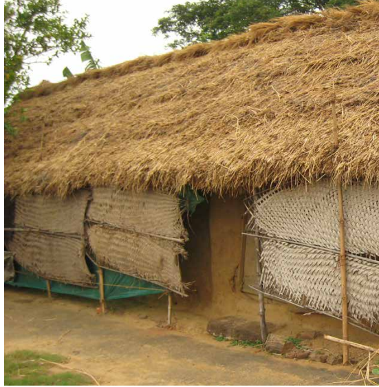
Fig. 21 (above) Rural hut with mud walls, thatch roof and palm leaf screens. Puri district, Odisha. Photo: AK.
