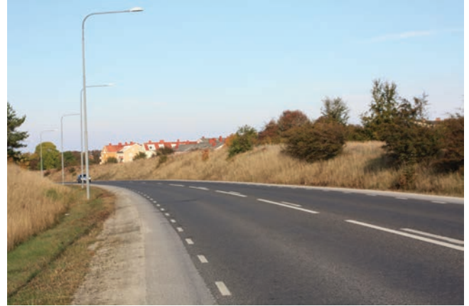
Färjeleden and its embankment along the north side. Photo (xxvii): Annie Lovén
