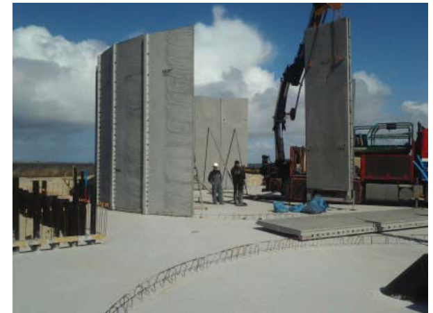
Above: Building the tanks that will hold adult salmon.
