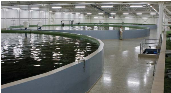
A typical hall with no daylight inlets to prevent algae from developing.
