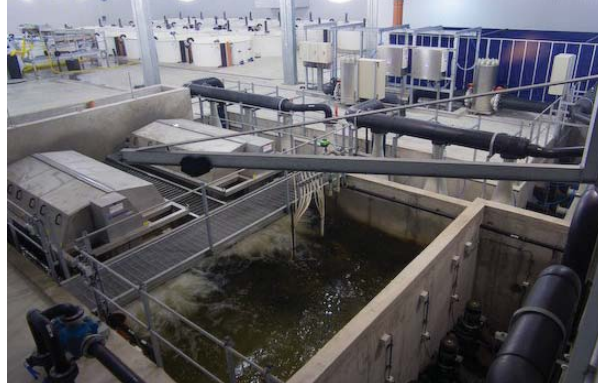
Filter and cooling plant for filtering intake water.
