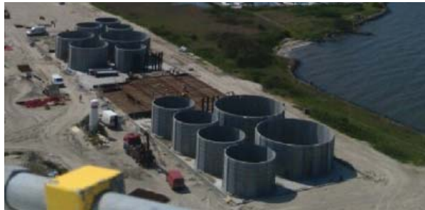
Above: The tanks of the Langsand plant in Hvide Sande, Denmark. The biggest are 25m in diameter.
