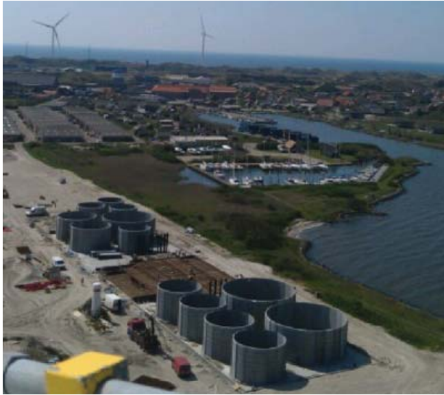
The plant in its entirety with it's tanks ranging from 15 to 25 meters in diameter.
