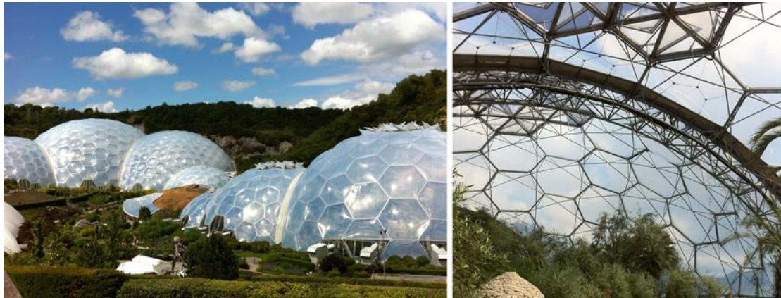
Figure 2.15 Eden Project in Cornwall by Grimshaw Architects and Anthony Hunt Associates. Eight large inter-linked domes create humid and temperate regions. The structure is covered with triple-layered pillows of ETFE foil, which was used instead of glass to create a light-weight roof structure (Eden Project, 2001).
