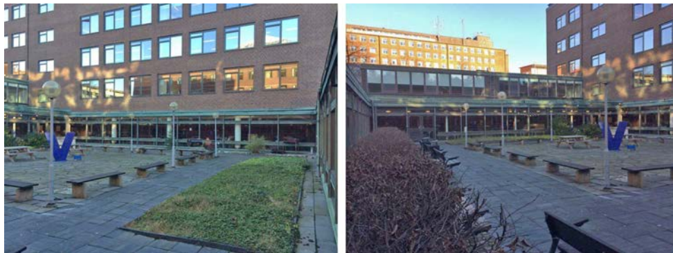
Figure 4.2 Existing courtyard at the civil engineering building, Chalmers University of Technology.
