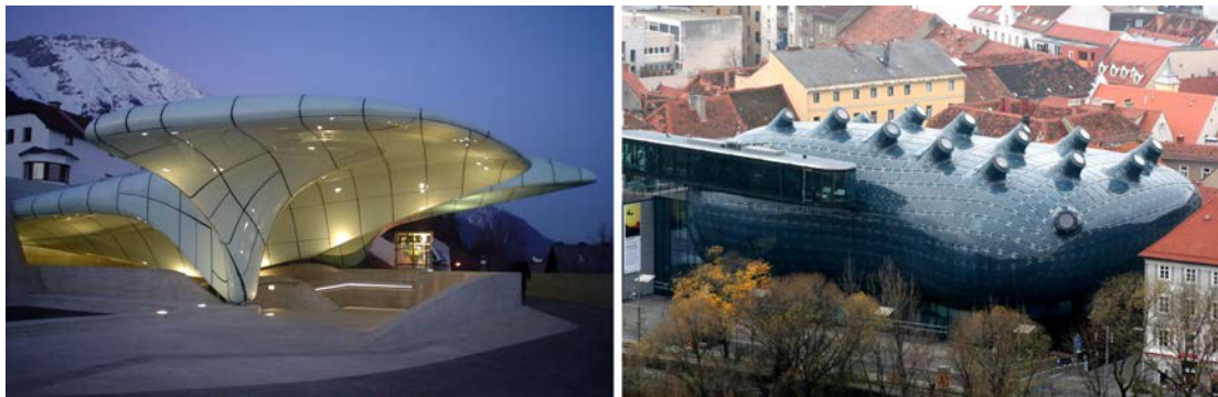
Figure 2.13 Left: Hungerburgbahn in Innsbruck by Zaha Hadid Architect (Photo: Hafelekar). Right: Kunsthaus in Graz by Peter Cook and Colin Fournier (Photo: Schneider & Aistleitner). In both buildings, a separate mould for each element was used.
