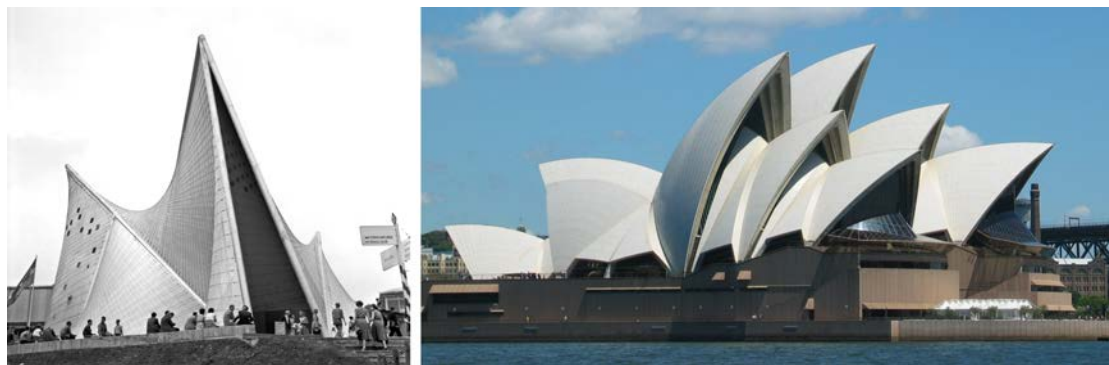
Figure 1.1 Left: Expo'58 pavilion Le Corbusier, 1958 (Photo: Wouter Hagens). Right: Sydney opera house, Jørn Utzen 1973 (Photo: Bjarte Sorensen). Both buildings got it's freeform shape realized by the use of reinforced concrete.
