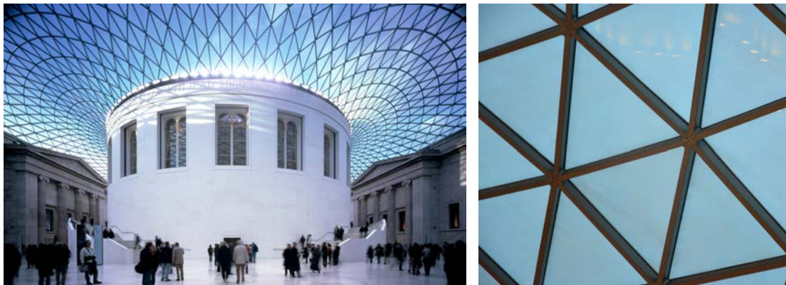
Figure 2.4 The Great Court of the British Museum in London is covered by glass with a triangular steel mesh. It was opened in 2000 and designed by Foster + Partners and Buro Happold.
