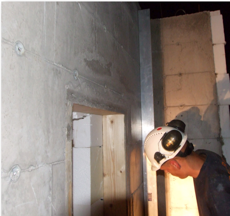
Figure 52: Verification with straight edge
