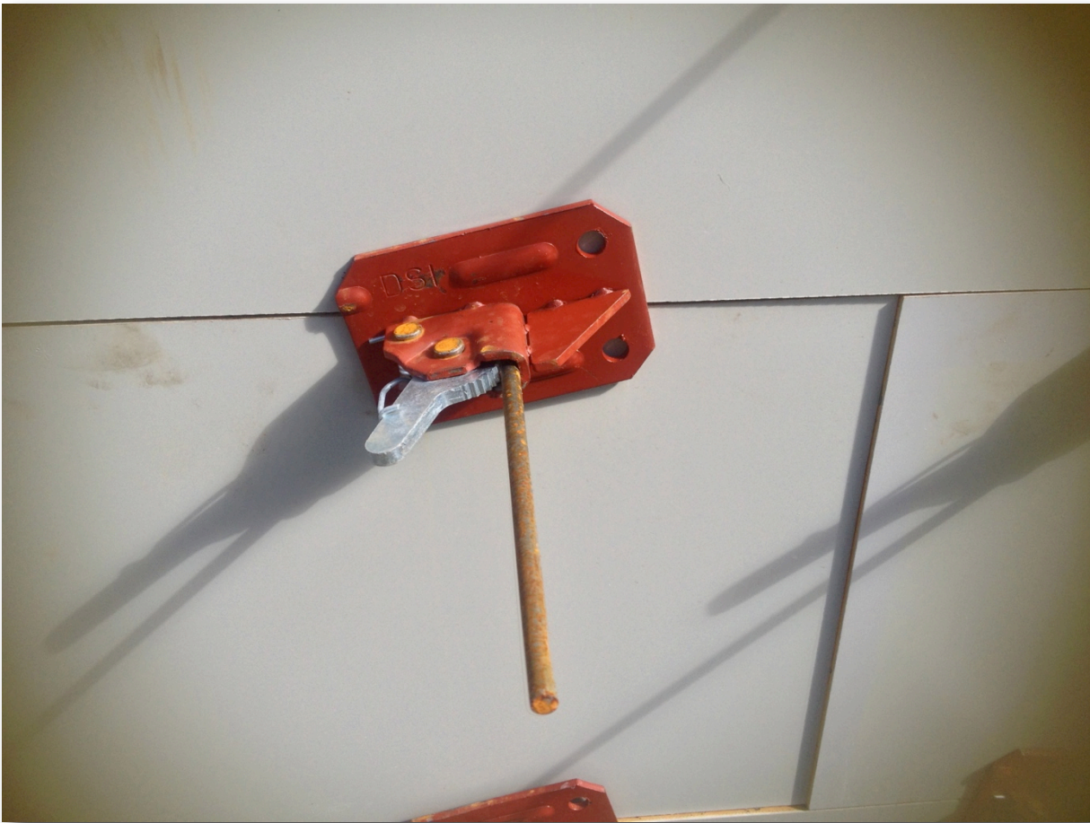
Figure 35: Mounted form lock with bad performance and the improperly aligned Sonoboards
