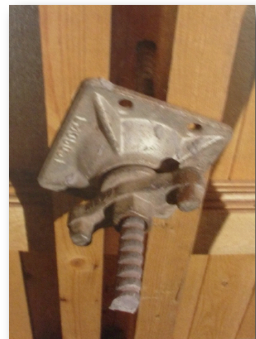
Figure 23: Form lock for wooden form
