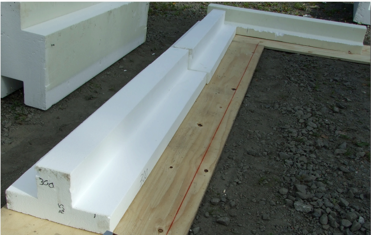
Figure 32: Styrofoam with a height to fit the Lower PUR.
