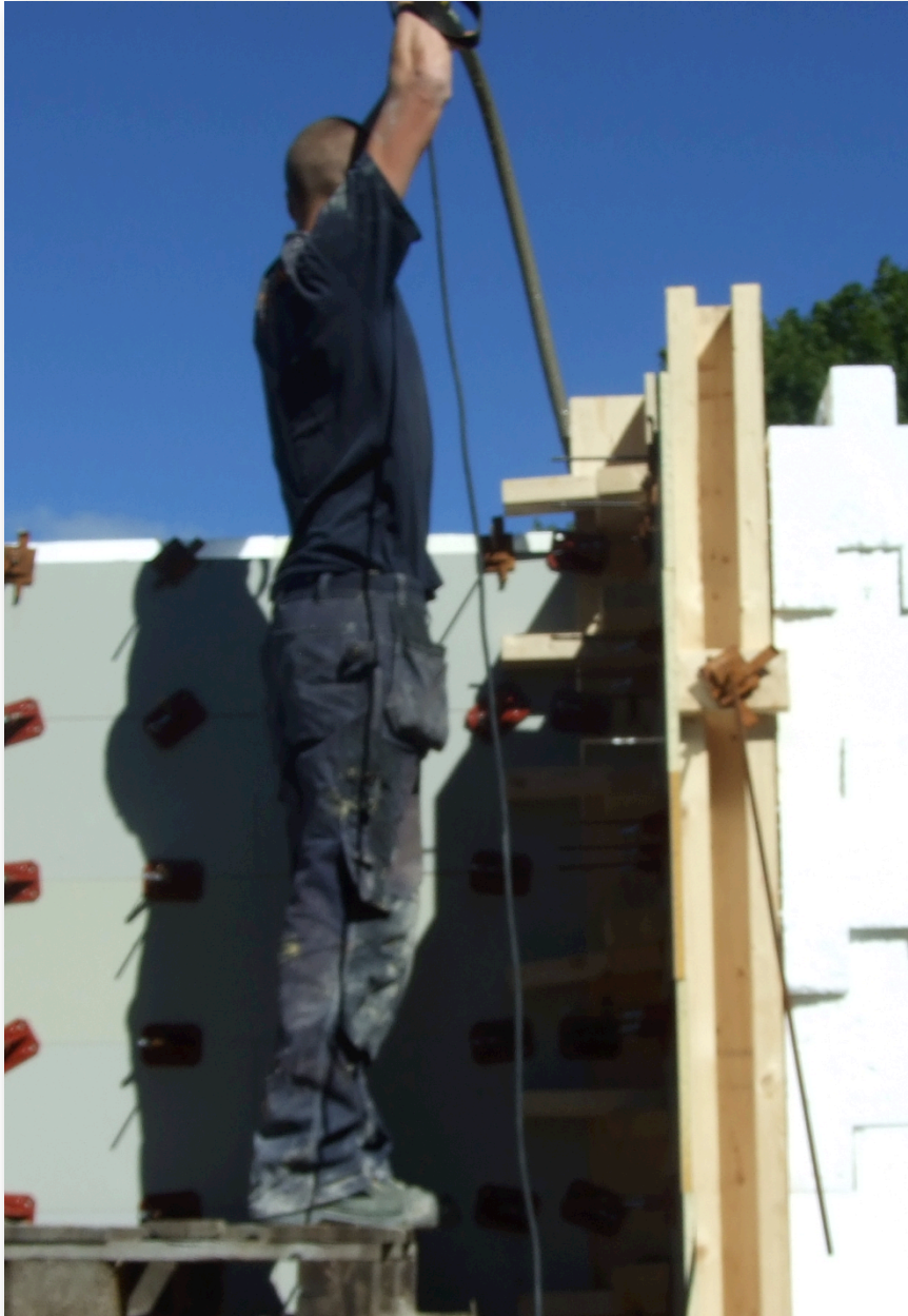
Figure 48: The vibrator is lowered into the form
