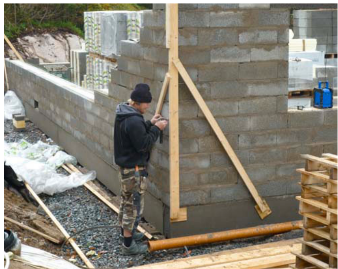
Figure 7: House built with Weber Isoblock (Weber, 2013)
