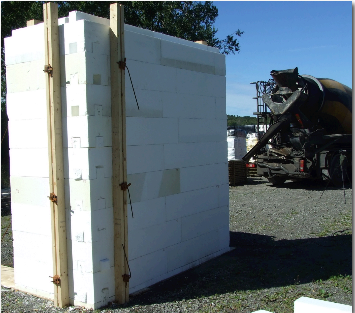
Figure 45: Wood studs on the back of the mould, each with 3 form locks that lock the 6 rebars on the inside of the mould.
