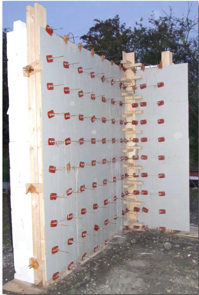
Figure 50: The mould before removal of the Sonboards
