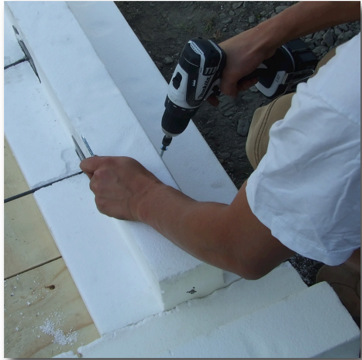
Figure 31: Screws through the Styrofoam into the plywood
