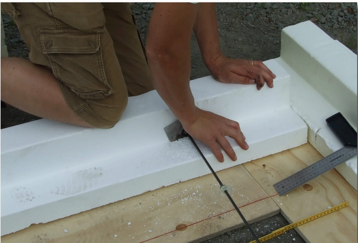
Figure 34: Mounting of form tie
