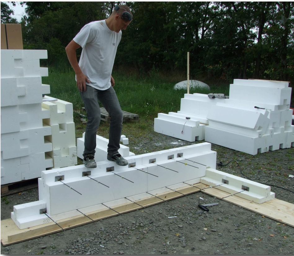
Figure 38: First layer of Styrofoam and form ties. The fit was really tight, so some parts needed to be exposed to a large force to place them in the correct positions.
