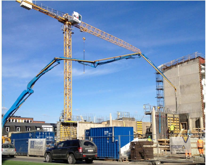
Figure 10: Construction site with crane and concrete truck
