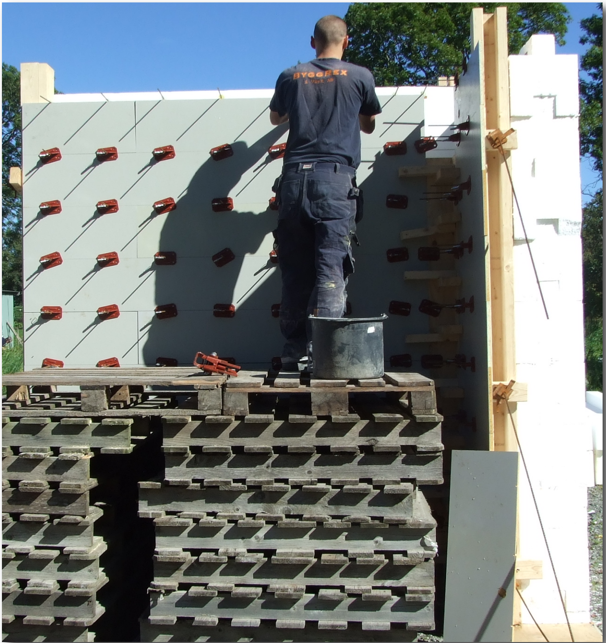
Figure 46: Mounting of the last form locks
