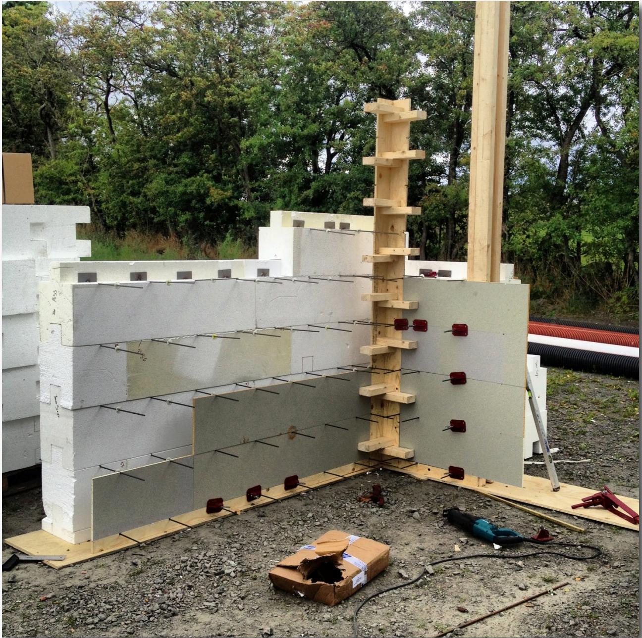
Figure 42: Test rig with corner solution and the wood stud that closes the right side of the mould.
