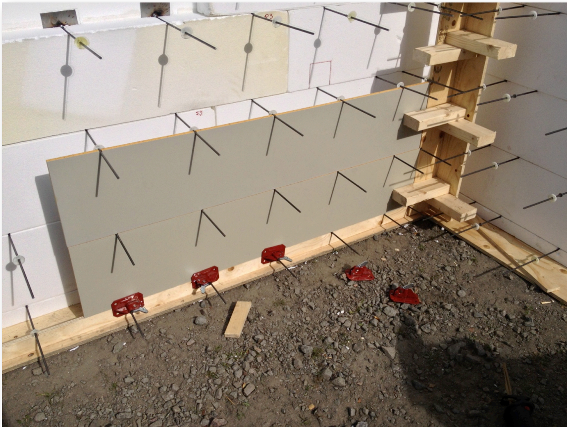
Figure 41: The first mounted Sonoboards and form locks.
