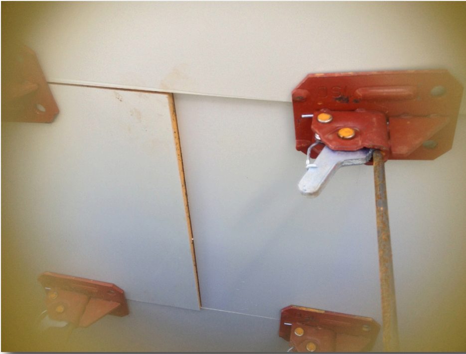
Figure 51: Malfunction form lock and deviating Sonobords
