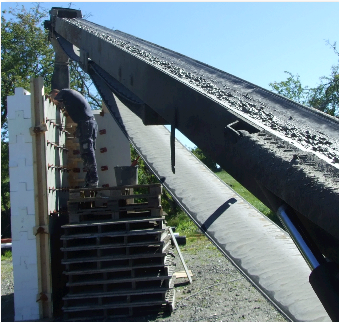
Figure 47: Pouring of concrete
