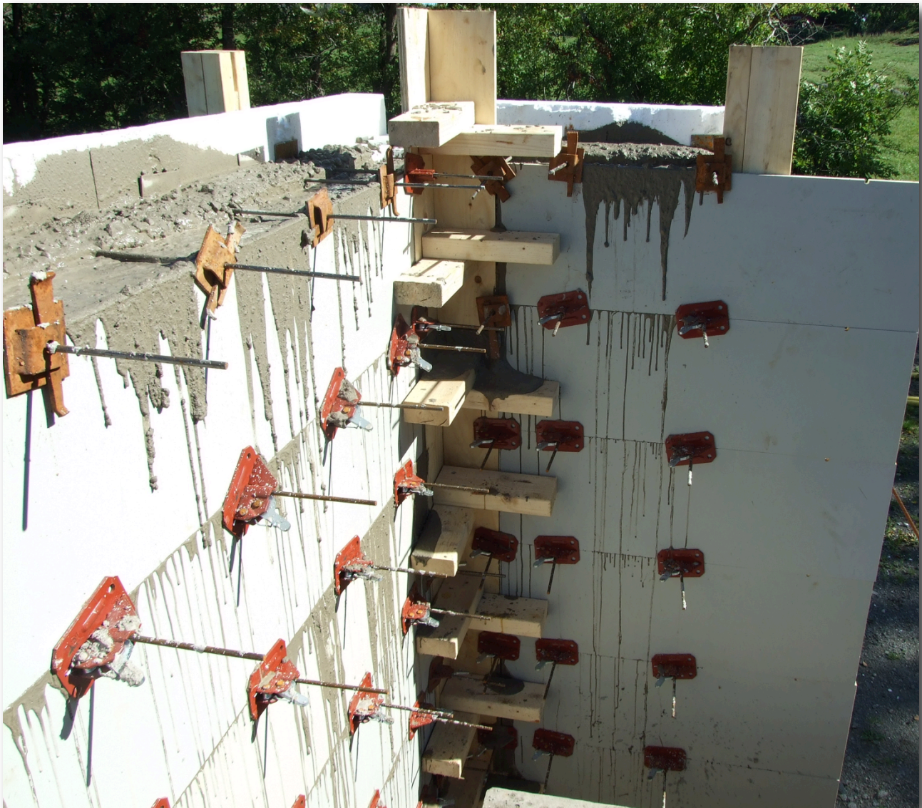
Figure 49: The mould right after the pouring of the concrete
