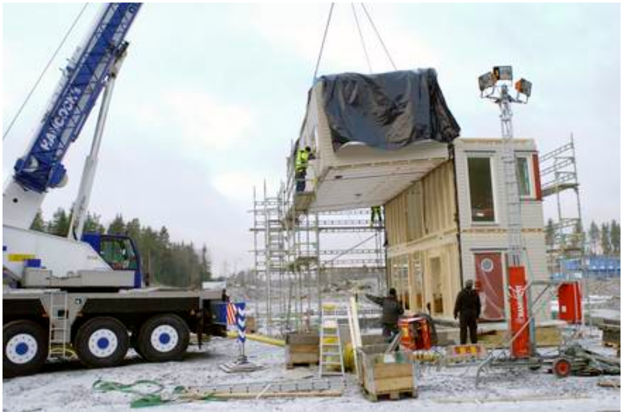
Figure 9: Prefabricated walls (Finndomo, 2013)
