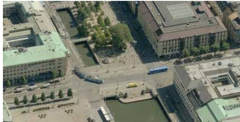
FIGURE 6.37 (Source: Google) The existing Brunnsparken
