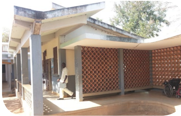
Rainwater is directed to the ground inside the pillars.
