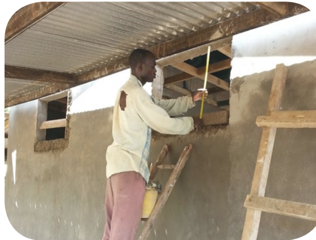
The holes for the small windows were adjusted.
