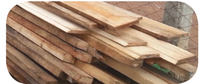
Roof structure : wooden trusses
