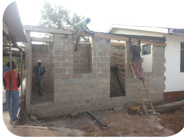
8. The wooden frames for the ring beam of steel reinforced concrete is taken down.
