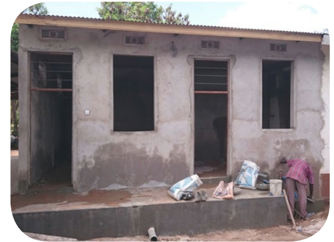
21. An inspection chamber for the plumbing is made, and the ceiling boards have been put up.
