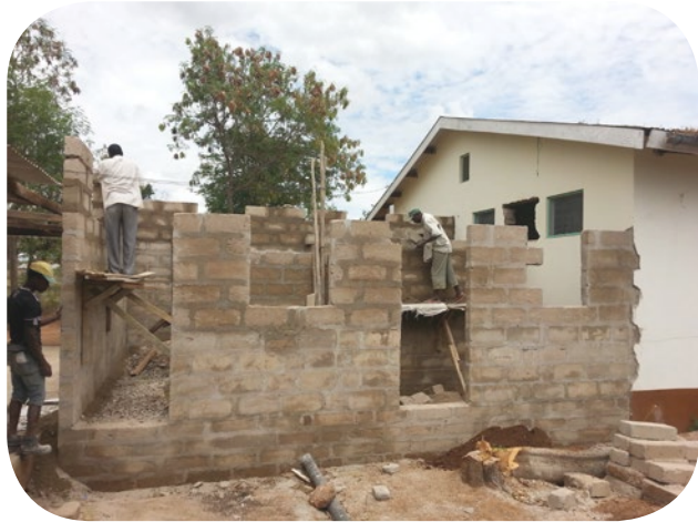
7. The walls are higher and the AC in one of the existing windows is removed.
