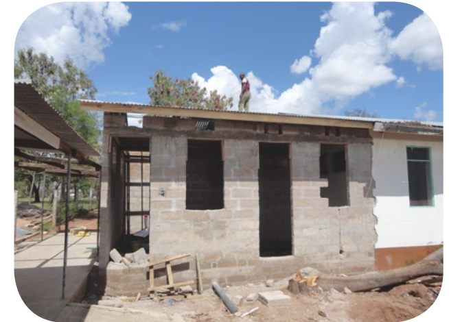
12. The iron sheets and the gutter boards are put up.
