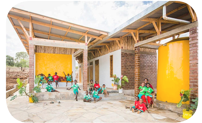
The water tank is integrated in the design.
