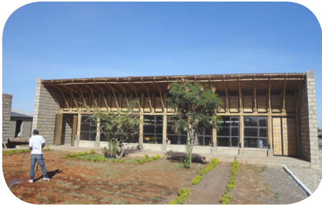
The roof is made of bamboo from Kenya.
