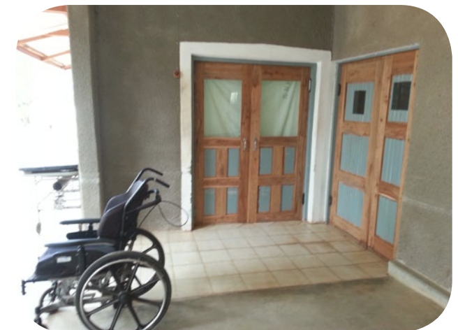
Two of the three doors we renovated, before painting.
