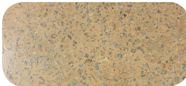
Floor: polished concrete floor with exposed aggregate
