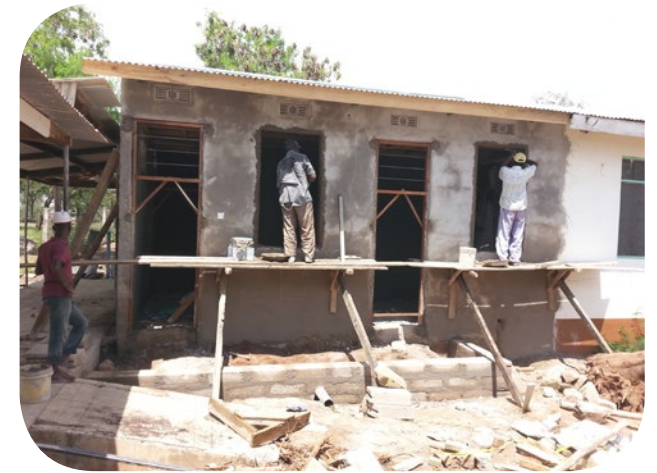
18. The corners for the windows and doors are plastered to look good.
