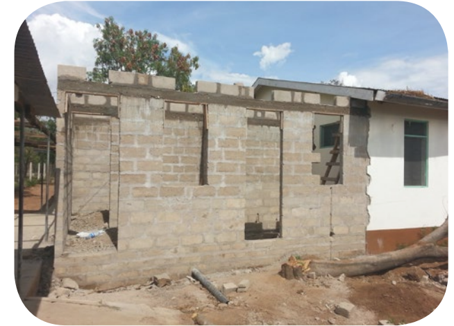
9. Another layer of bricks above the ring beam. Holes for the plumbing were made.
