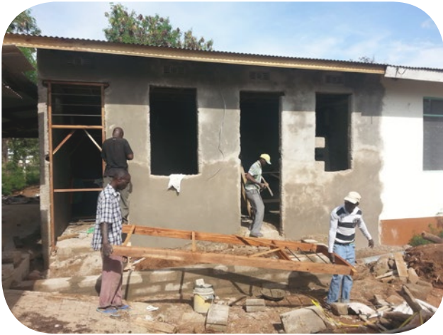
16. The wooden frames for the doors are installed, and so are the switches for internal and external light.
