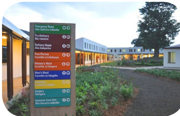
There are clear signs in the central courtyard. (c) MASS Design Group
