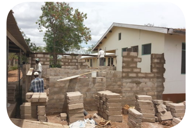
A maternity theatre extension through joint efforts.
