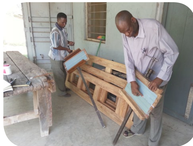
The inner parts of the old doors are reused.
