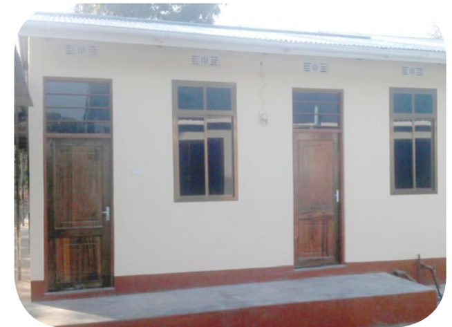
24. The building is painted.
