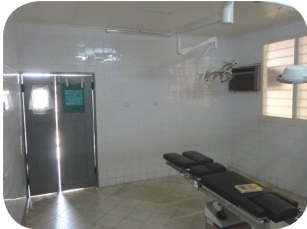
The door gap lets air and dust enter directly into the theatre.
