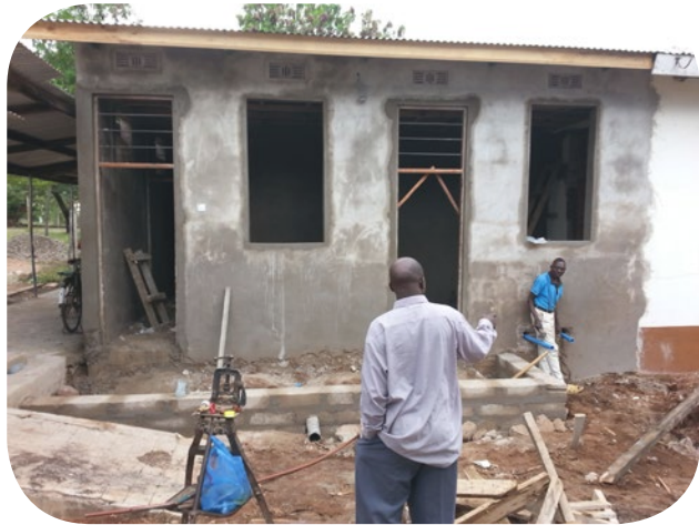
19. Pipes for the water and plumbing are installed.
