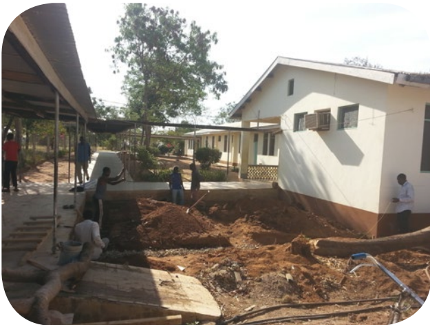
4. Digging for the foundation.
