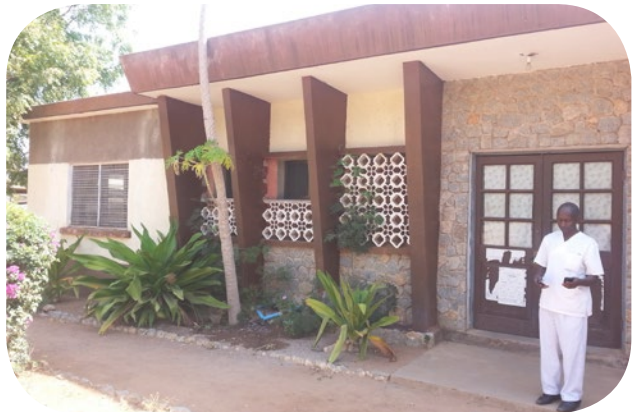
The infusion unit is in the old administration.
