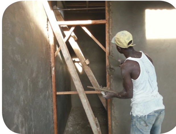
Plastering around one of the door frames.
