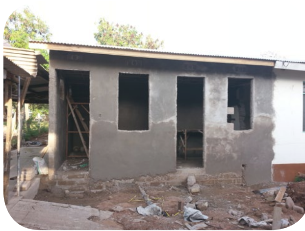
17. The inclination of roof over the path to the left was changed to direct rainwater away from the building.
