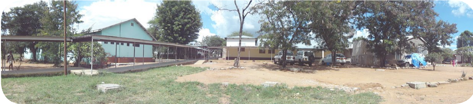
This panorama is taken from the kitchen building. The eye ward is in the green building to the left. The building at the far end is the pharmacy. To the left in the grass you can see an inspection hole for the main water line that passes from right to left in the picture.
