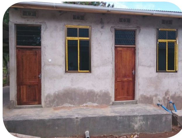
23. The doors are varnished and glass installed above the doors.
