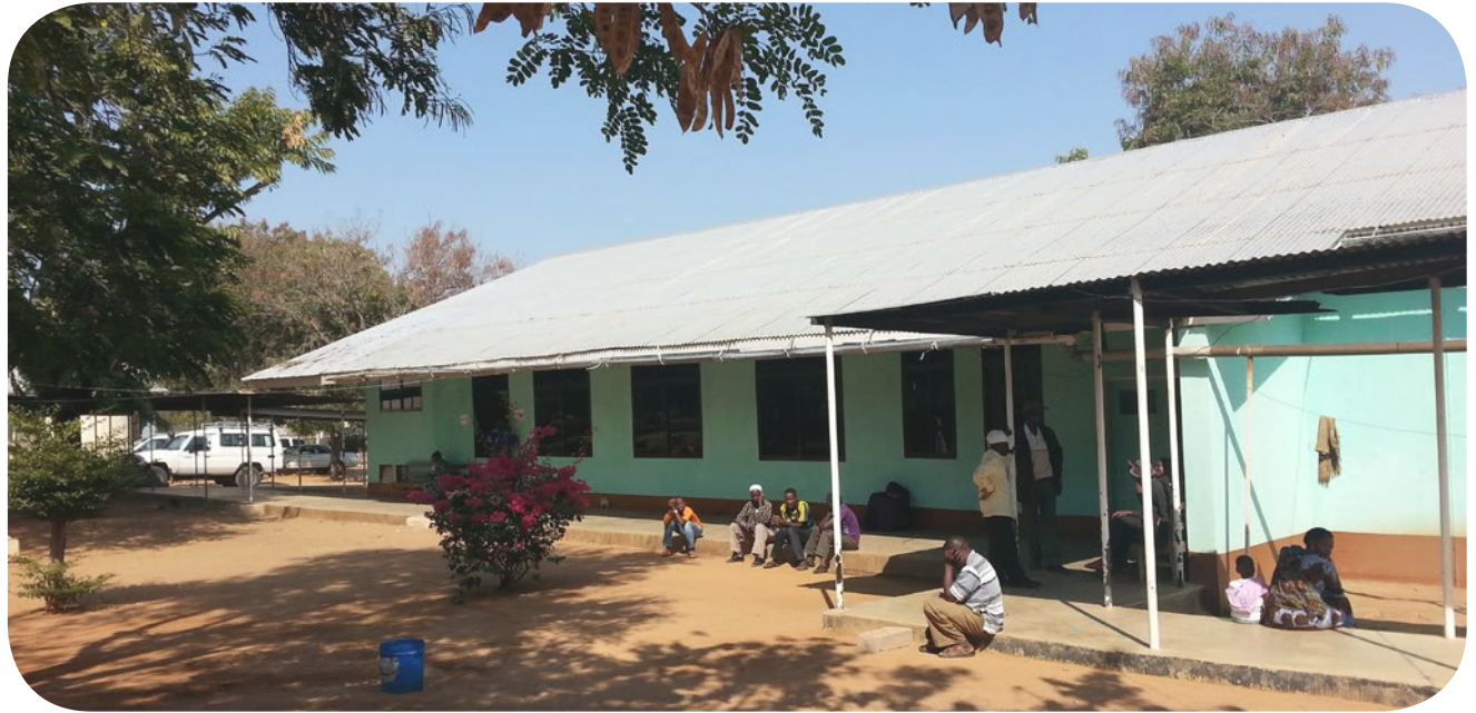
The existing building for the eye clinic and the eye ward.
