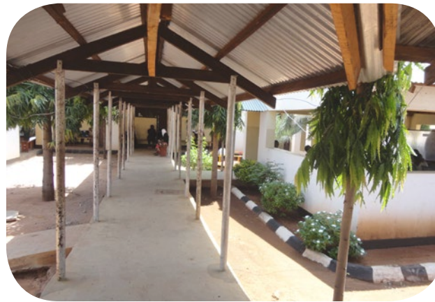
The outdoor walkways at Shinyanga Regional Hospital.
