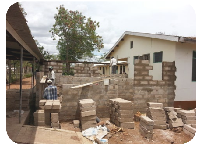
6. The walls are coming up and one can start to see where the windows and doors will be.
