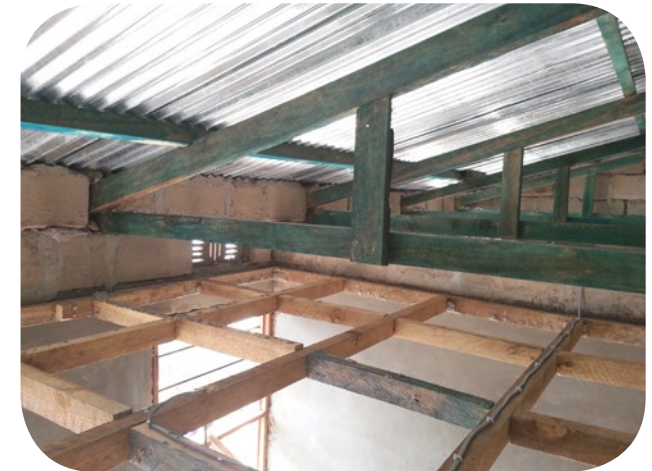
The roof is ventilated between the roof and the ceiling.
