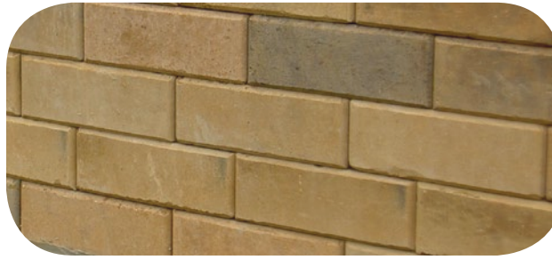
Walls: interlocking compressed soiled blocks (Makiga Engineering)
