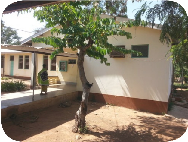
1. The site for the extension. The existing theatre is just inside the wall.
