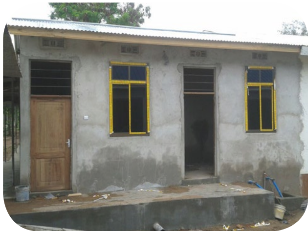
22. Wooden doors and aluminium framed windows are installed.
