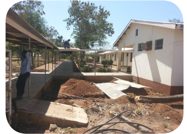
3. The roof over one of the paths is taken down and the water pipes crossing the site are being moved.
