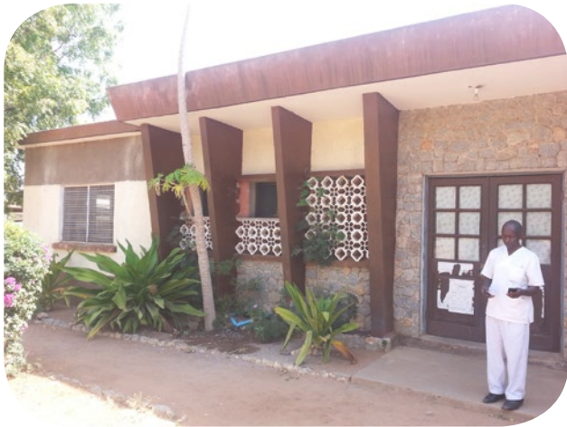
The infusion unit is in the old administration building from 1961.
