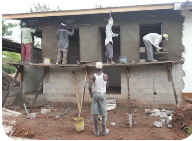
14. Plastering the walls.
