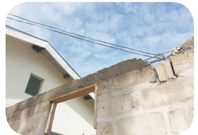
At the construction site.
