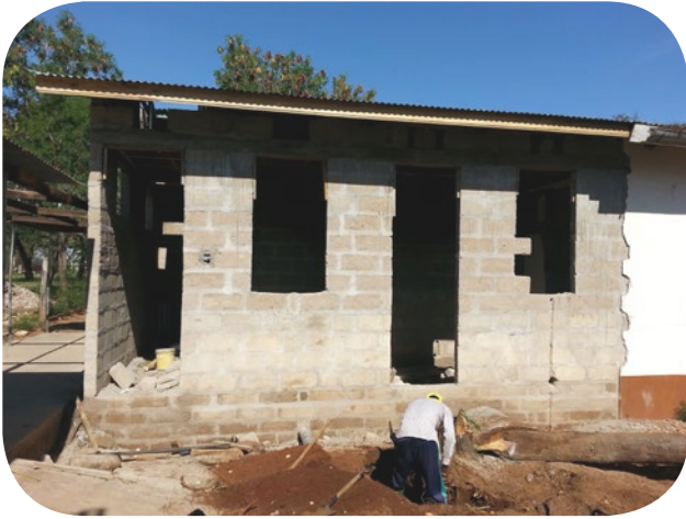
13. The stump of the tree is removed and the ground smoothed in preparation for the new path to be built.
