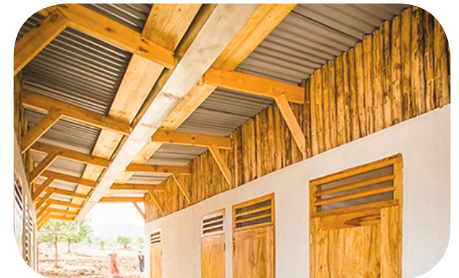
The roofs are leaning to the middle of the building where the rainwater is collected in a gutter.
