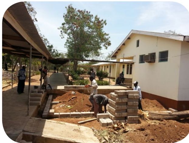
5. The first cement blocks have been places and the craftsmen are double checking the measurements.
