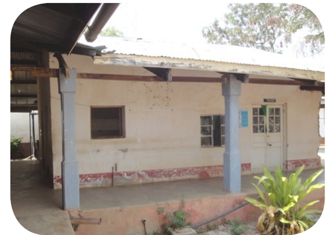
The physiotherapy building is in a poor condition.
