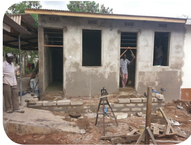
20. The cement floors are made, and one more layer of brick is added for the new path.
