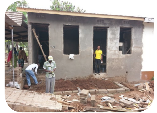
15. Building the new path for the entrance doors, at the same time as electrical wiring is going on.
