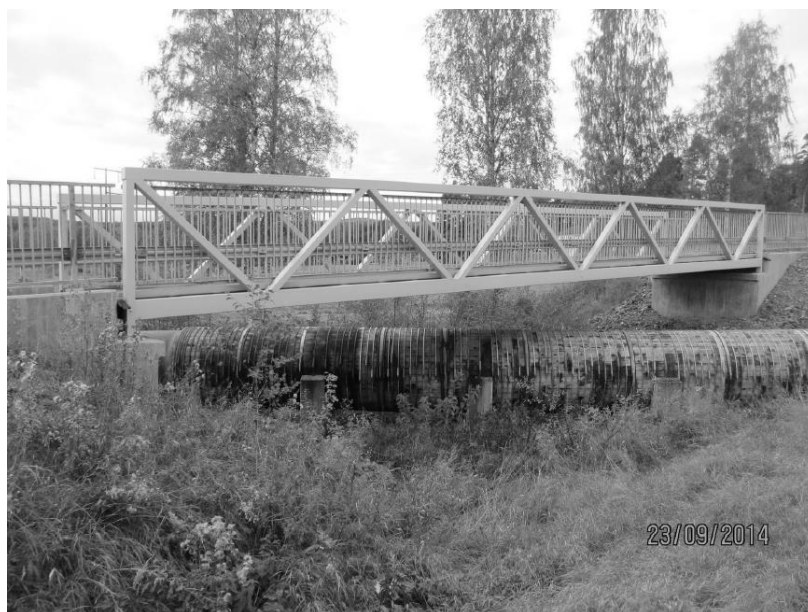
Figure 6.2 The steel bridge (BaTMan 2015b)
