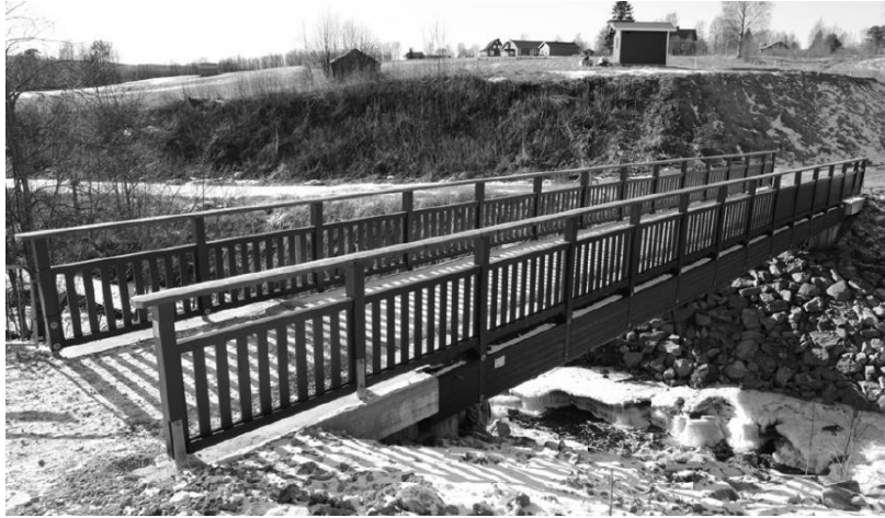
Figure 6.1 The timber bridge (BaTMan 2015)
