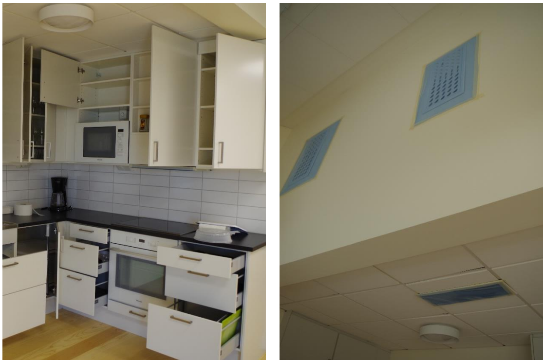
Figure B.1 Preparations for the Co-heating test.
