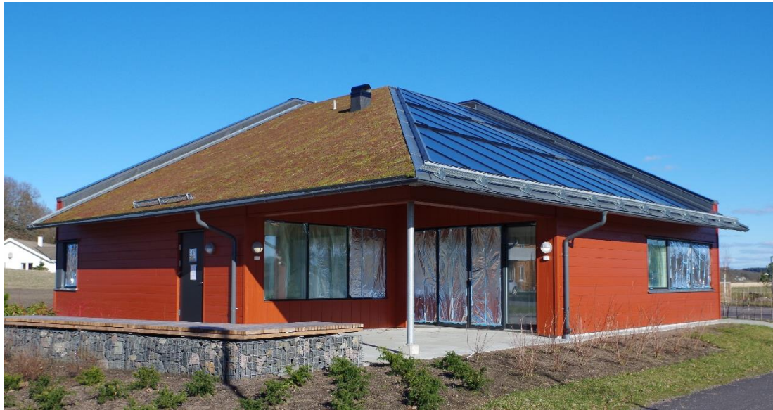
Figure 7.1 Community Building in Vallda Heberg where measurements are performed.
