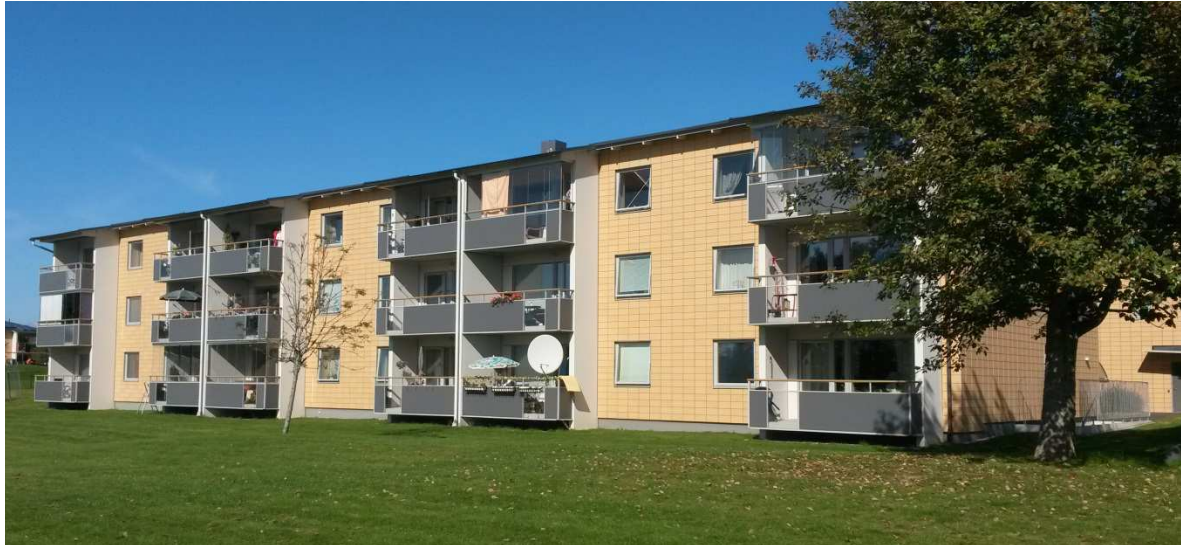
Figure 6: House K after extensive renovations.
